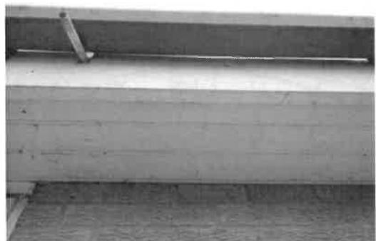
The loft space is insulated and roof tiles are lined with a modern breathable membrane.
