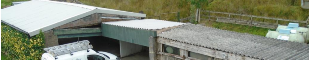
Garage and shed roofs
