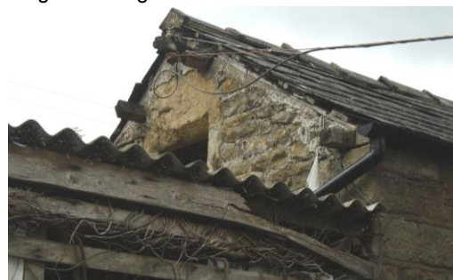
outbuilding gable and part shed roof
