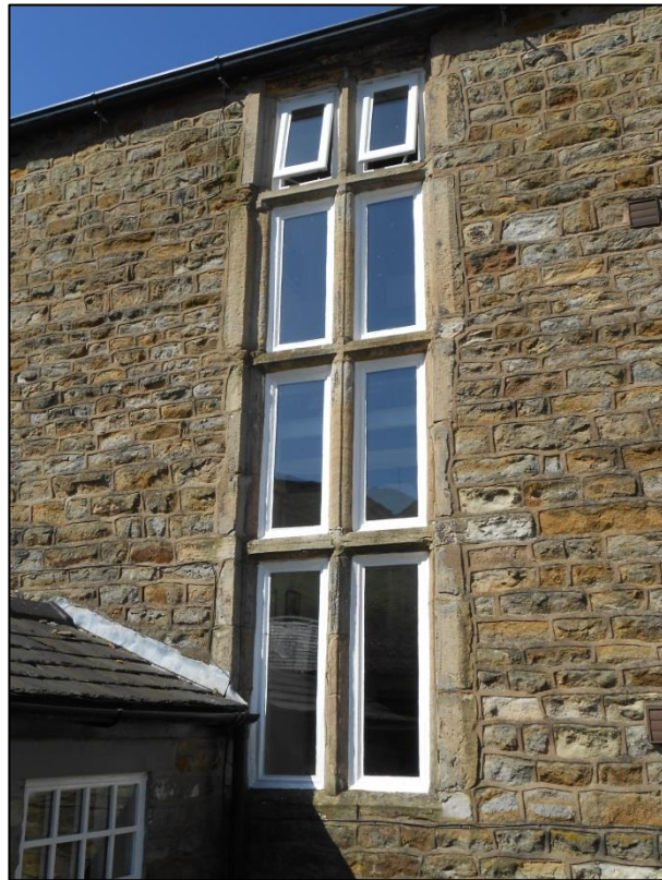
PL00: Existing staircase window present to the rear east facing elevation
