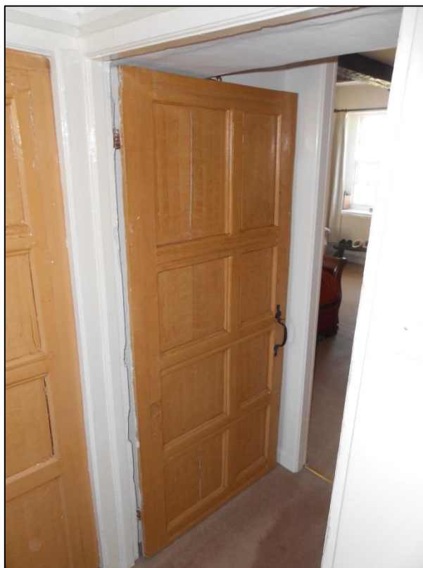
PL00: Original internal door present to the first floor of the building to the front south west bedroom
