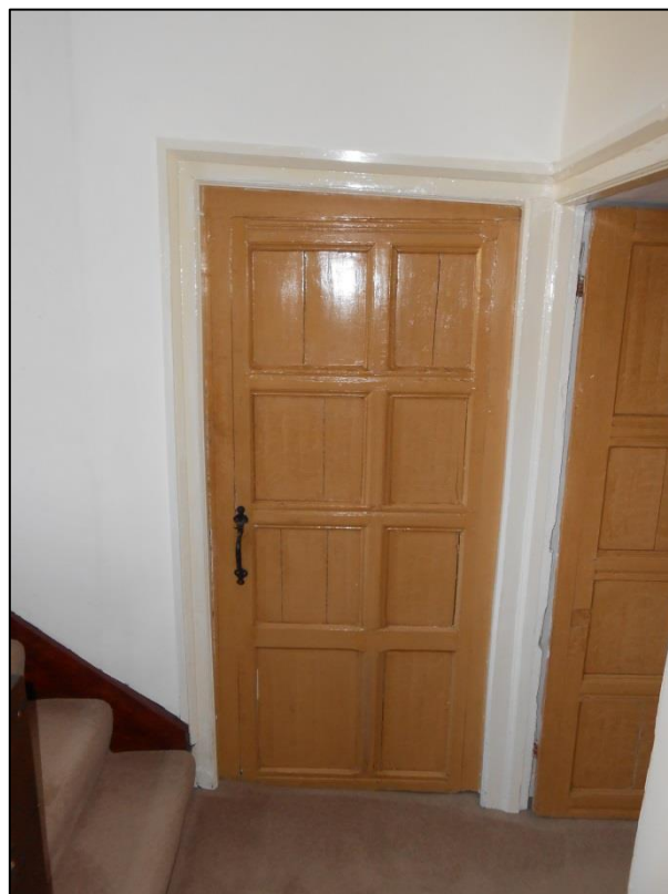
PL00: Original internal door present to the first floor of the building (now fixed shut) to the south east of the building.
