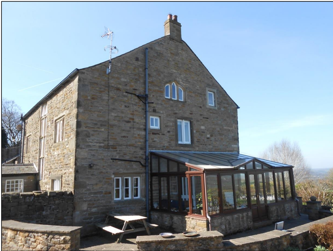
PL00: View of the building from the north
