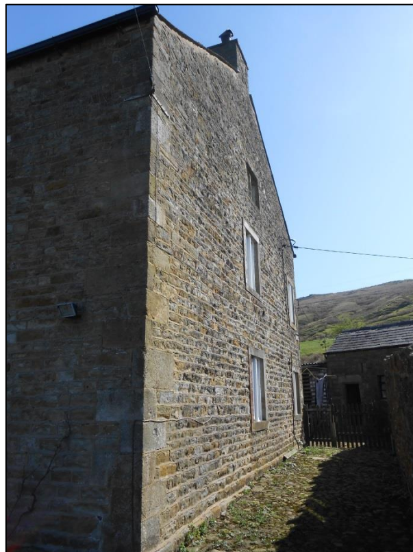
PL00: South facing elevation of the building
