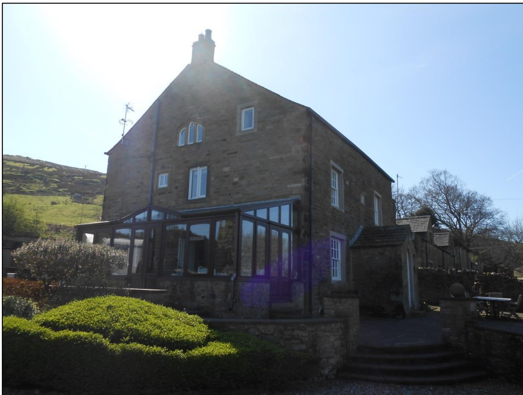
PL00: View of the building from the north west
