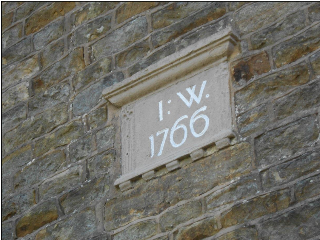
PL00: Date stone present to the front west facing elevation of the building.
