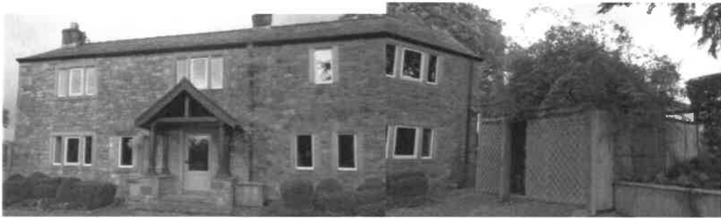
Front west elevation with porch
