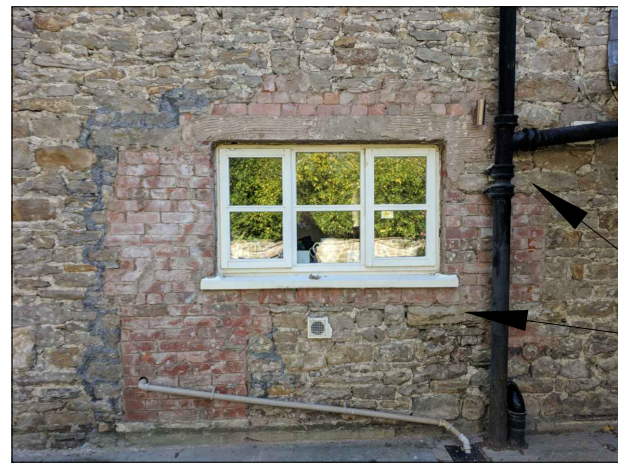
Existing lintel and cill in place where previous window was historically located
