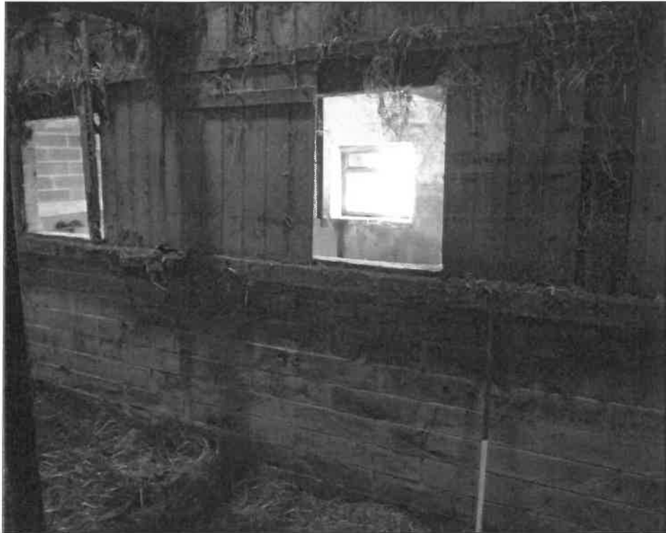
Plate 6. Bead-moulded sliding shutters, looking south-east, scale 1m
