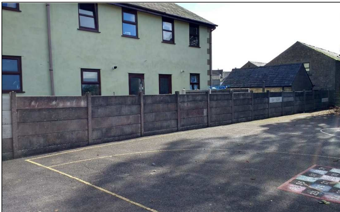
Figure 2: Existing Perimeter Fence at the South East Boundary (Fence Ref No.2 as per Drawing LPS/2017/001)
