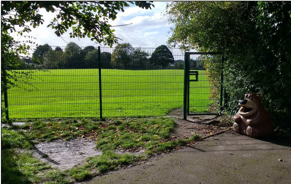
Figure 3: Existing Rear Fence at the Southern Boundary
