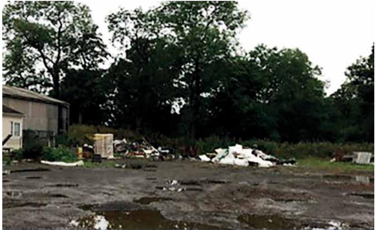
FIGURE 1: PHOTOGRAPH OF PART SOUTHERN SECTION OF APPLICANT SITE (EXCLUDING ACCESS TRACK)
