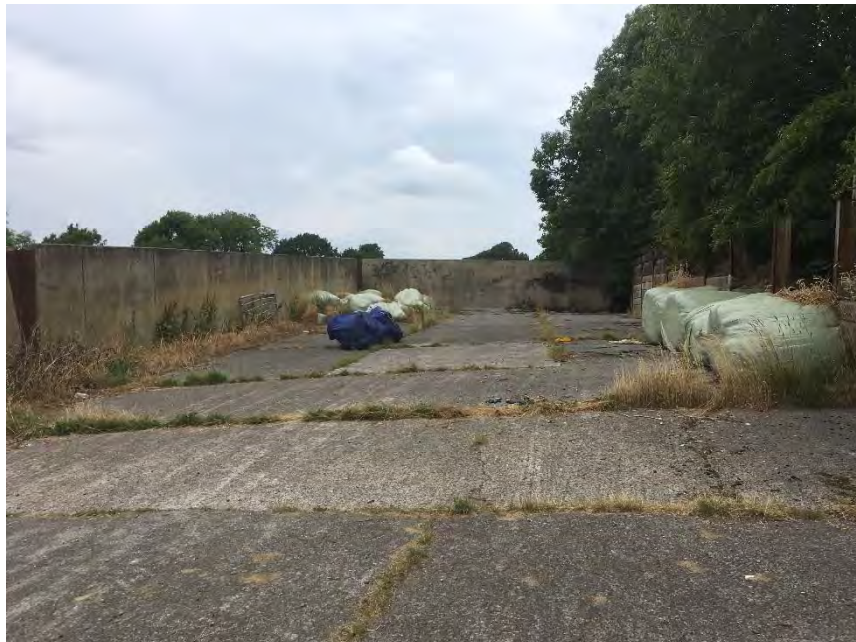
Photograph 8 – Area of concrete storage in the north-eastern corner
