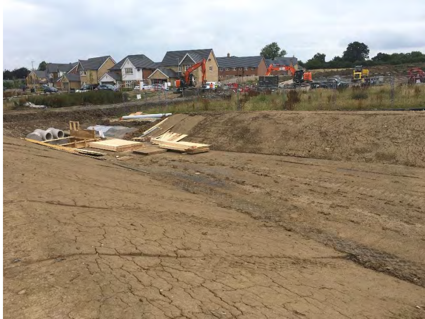
Photograph 7 – Construction area comprising partially built attenuation ponds and remnants of grass
