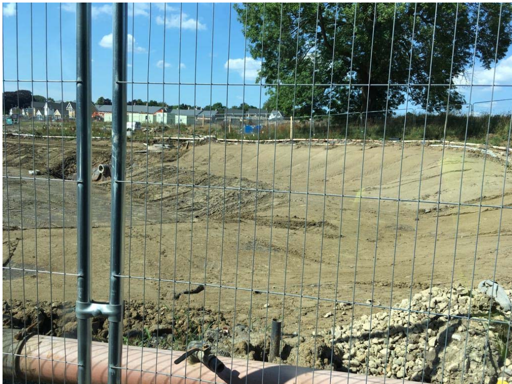
Photograph 2: Attenuation pond being constructed
