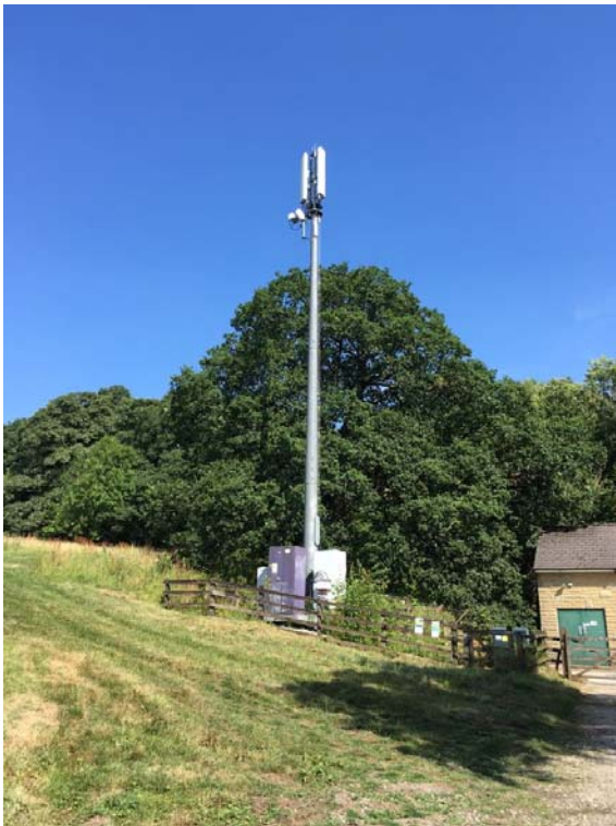
Photograph 4: Telecoms mast and United Utilities building
