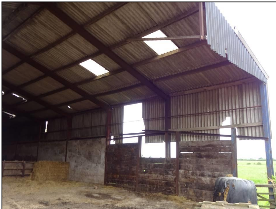
Photograph 4 showing the interior gable end of the Large Barn
