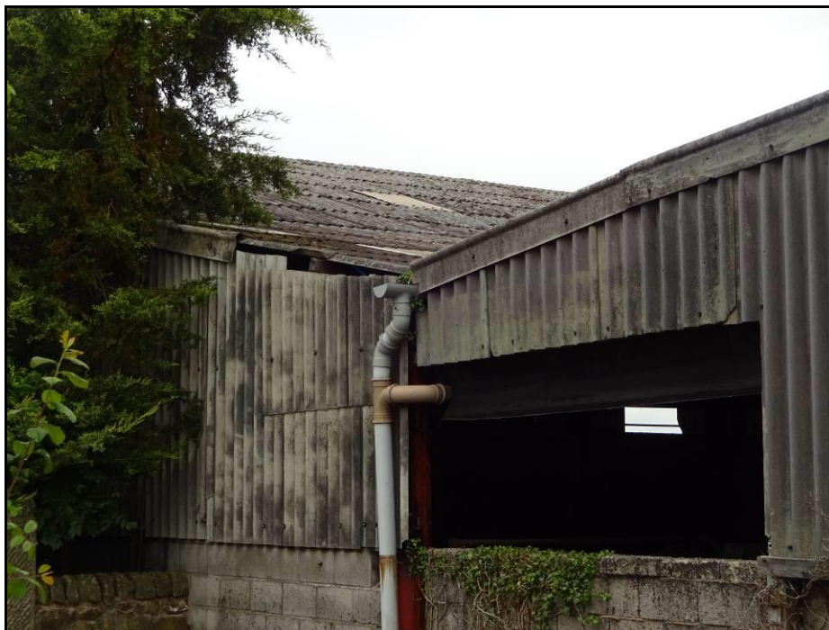
Photograph 2 showing the corrugated asbestos walls and roof
