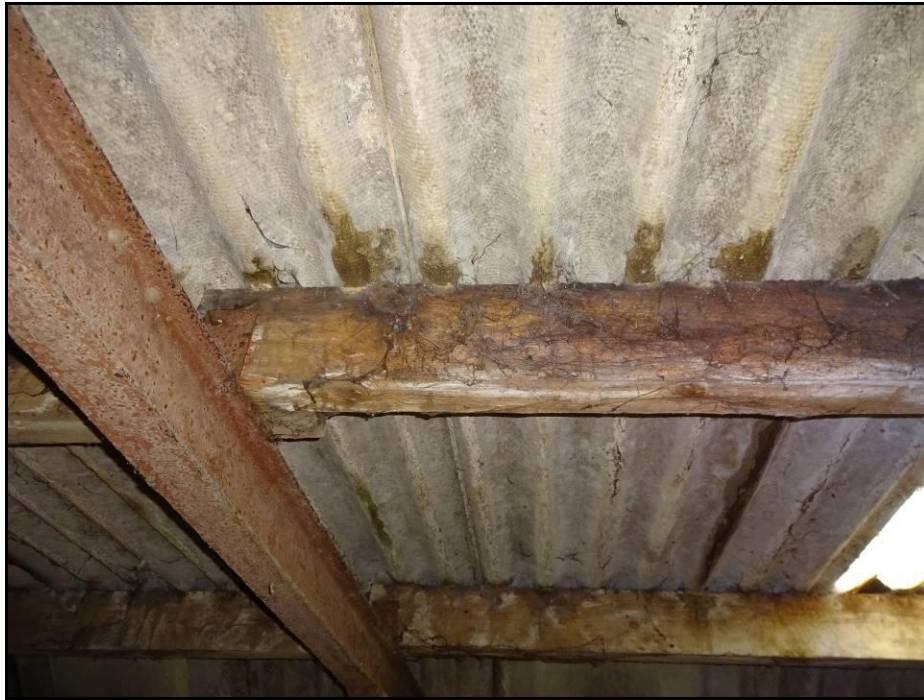
Photograph 11 showing the roof beams of the Feeding Shed
