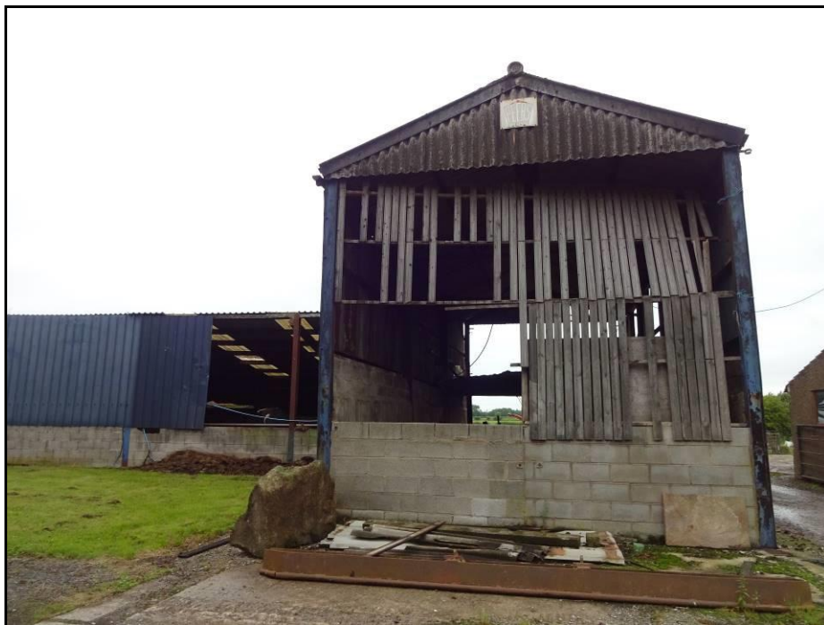
Photograph 5 showing the walls of the Small Barn
