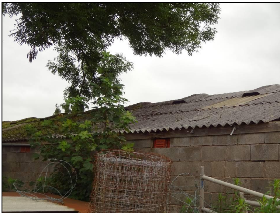
Photograph 10 showing the roof of the Feeding Shed from the north of the property
