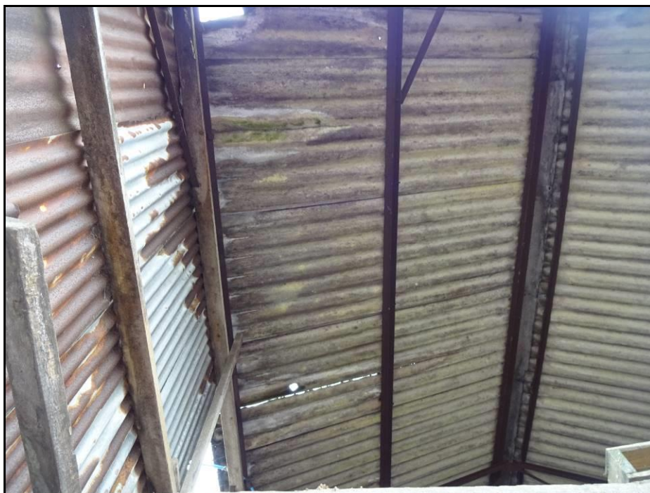
Photograph 7 showing the internal roof beams of the Small Barn
