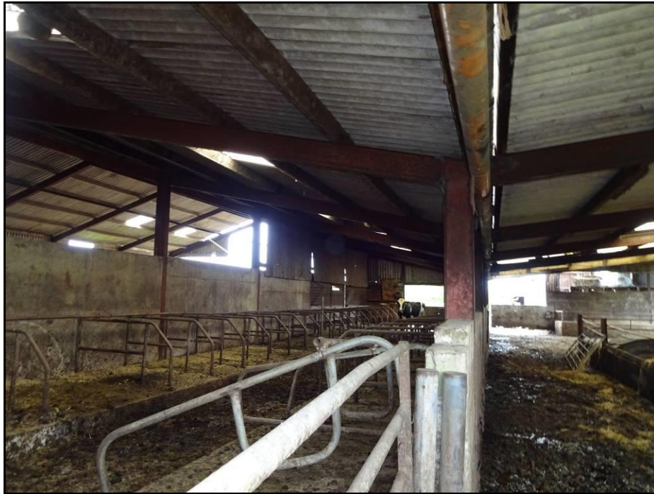
Photograph 3 showing the internal roof beams of the Large Barn
