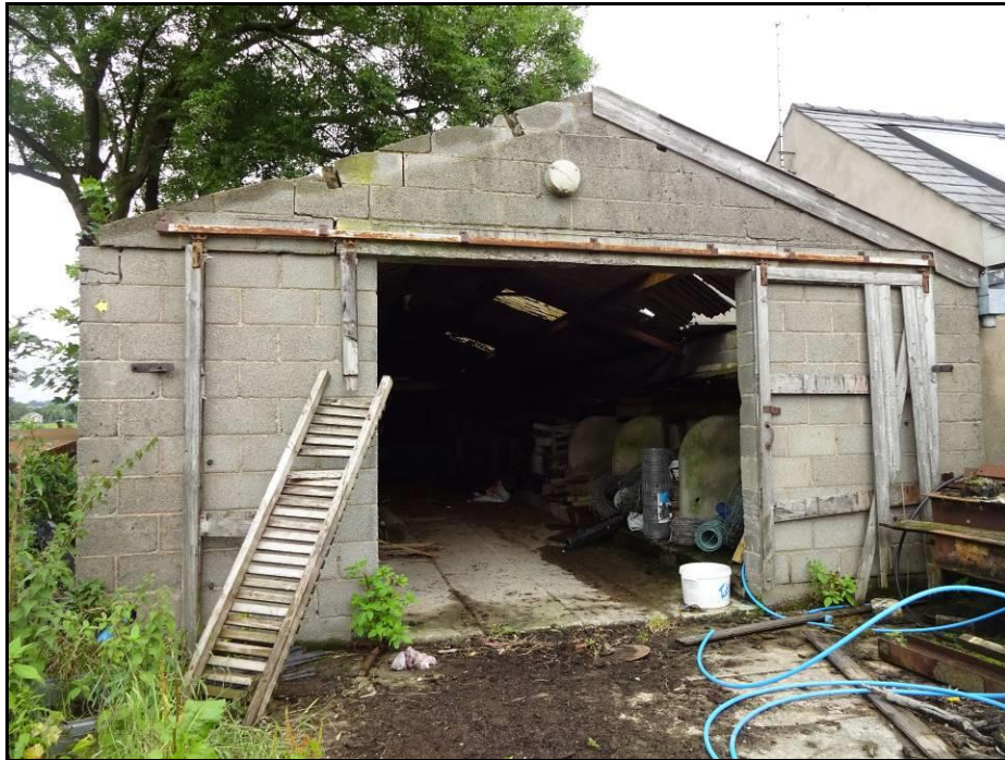
Photograph 9 showing the front of the Feeding Shed
