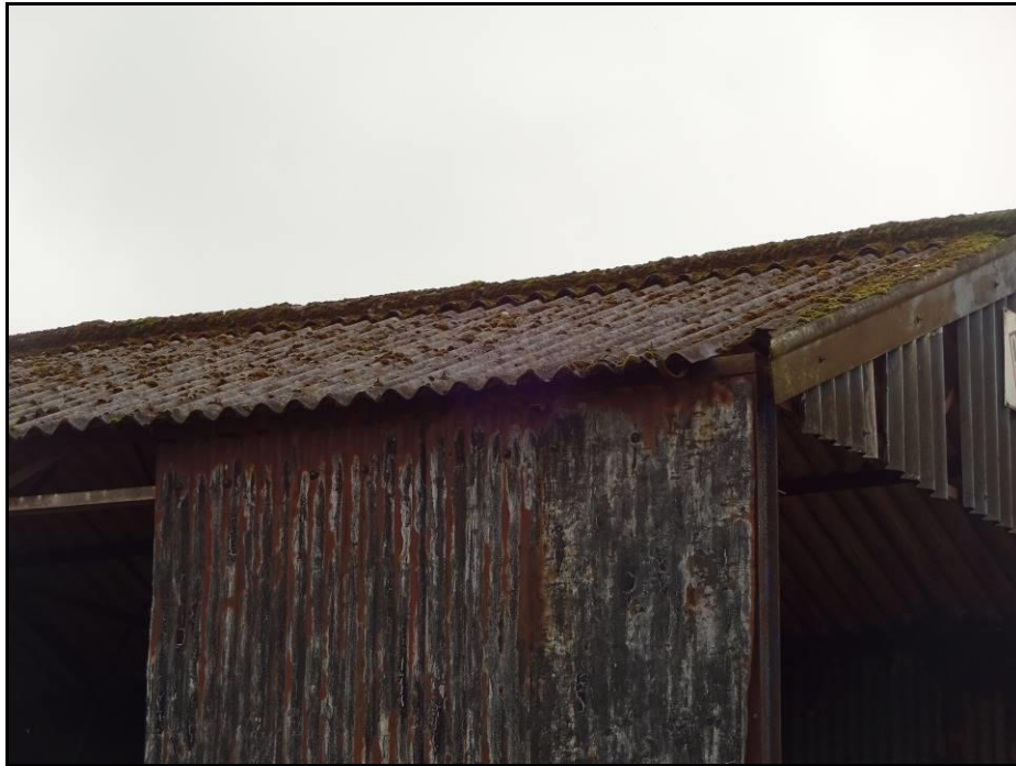
Photograph 6 showing the roof of the Small Barn
