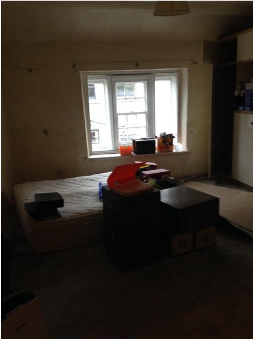
Figure 14 – 1 st floor, looking to front of premises
