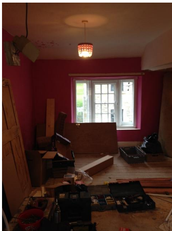
Figure 13 – 1 st floor looking to front of premises
