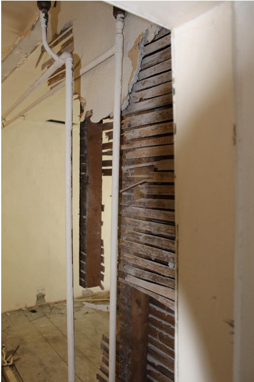
Figure 15 – Lathe and Plaster
