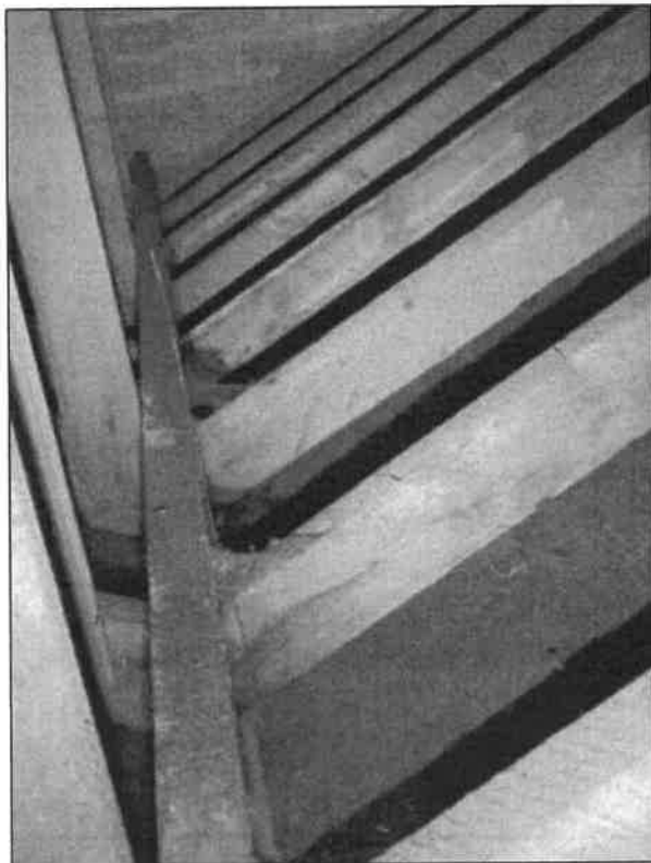
Plate 17: The northern aspect of the loft lacked any bat droppings and contained a greater number of cobwebs, suggesting bats were not using this area of the loft void.
