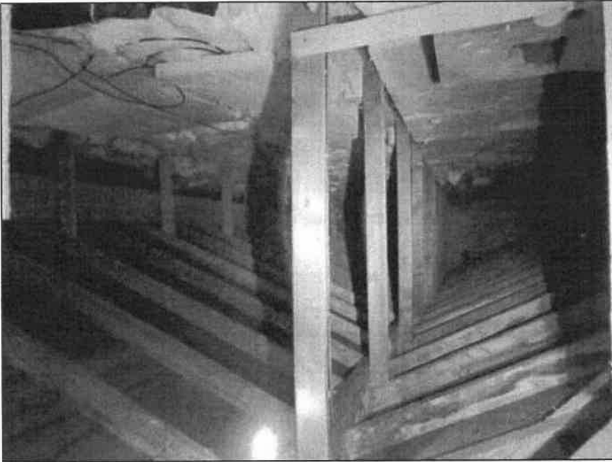
Plate 10: The loft void was warm, dark and well insulated.
