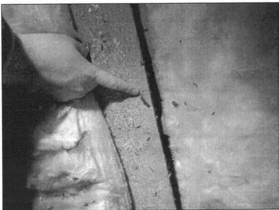
Plate 13: Directly beneath the ridge beam a number of droppings were identified throughout both the southern and eastern aspects of the loft void.
