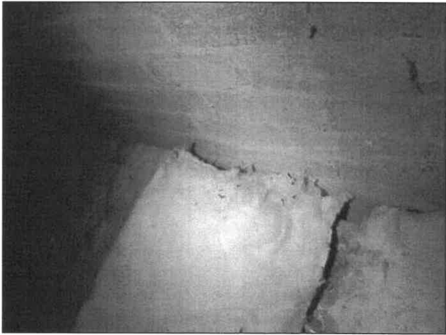
Plate 16: Droppings at the foot of the gable wall suggested bats were using this feature.
