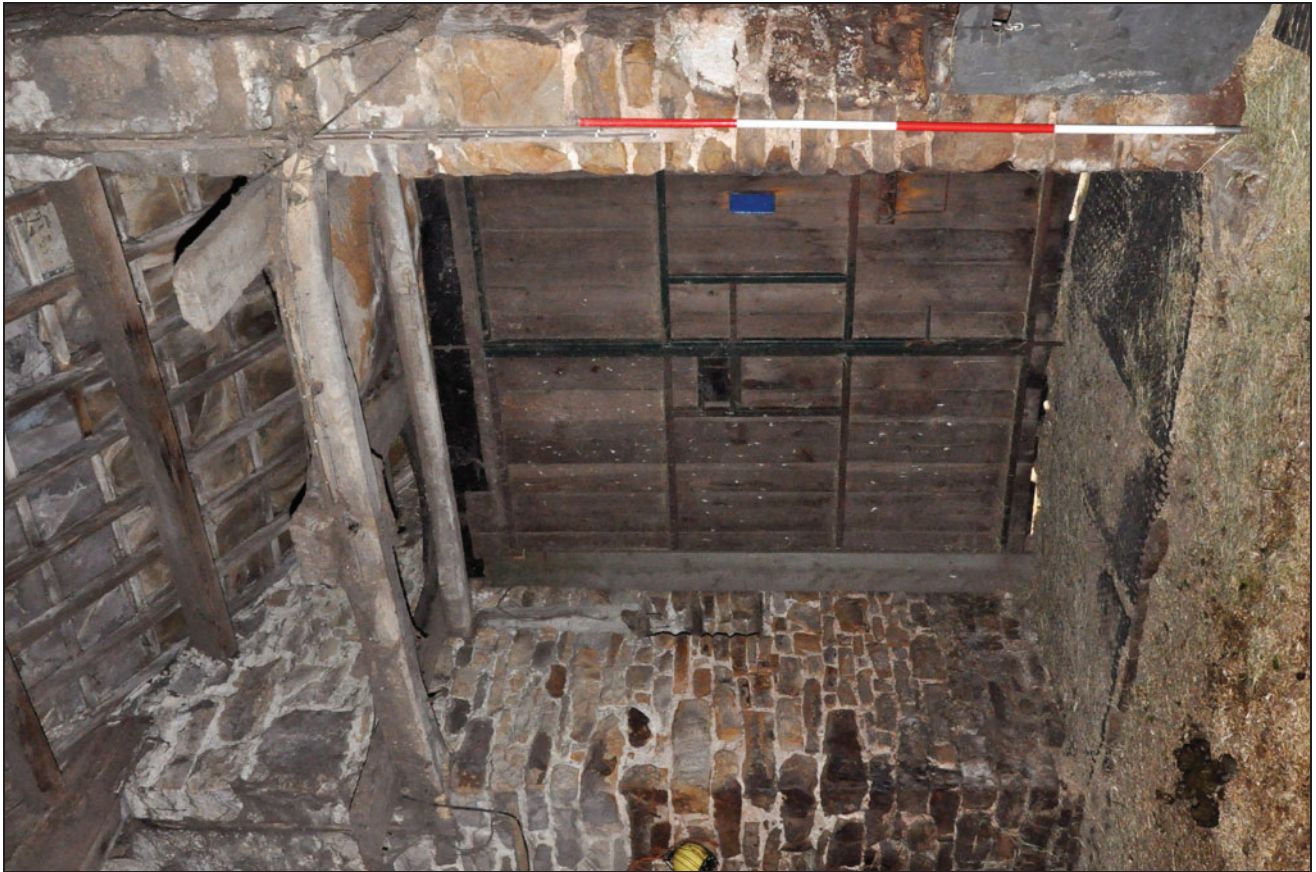
Photo 5: Internal view of porch, looking east
