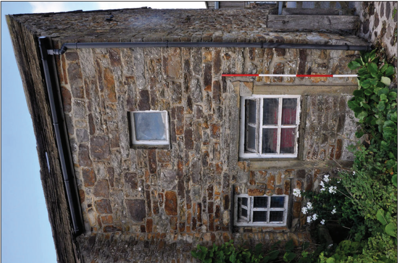
Photo 11: North-east end of front elevation (former doorway to stable?)
