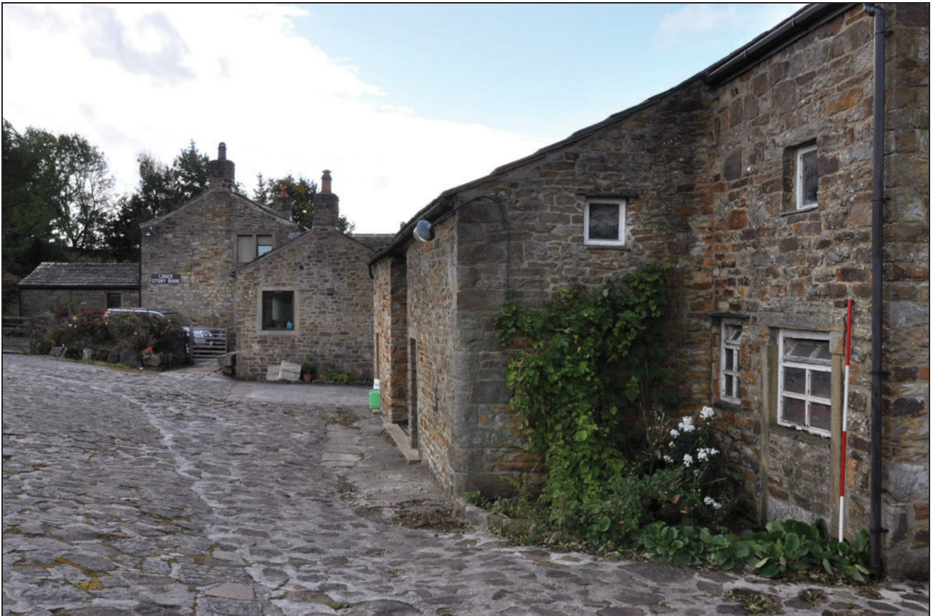
Photo 2: Barn and farmhouse, from the north-east
