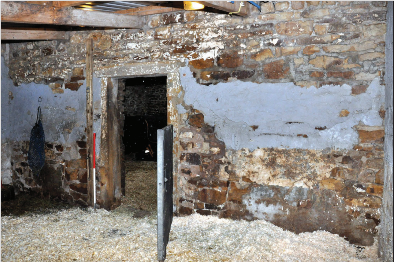
Photo 15: Detail of altered doorway in rear elevation, now within lean-to
