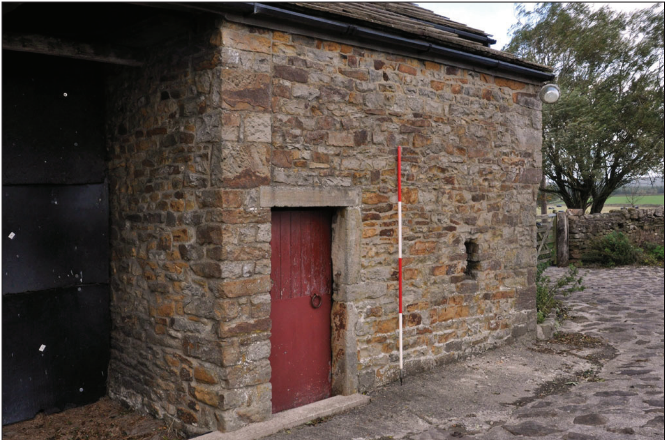
Photo 8: Historic addition to front elevation, looking north
