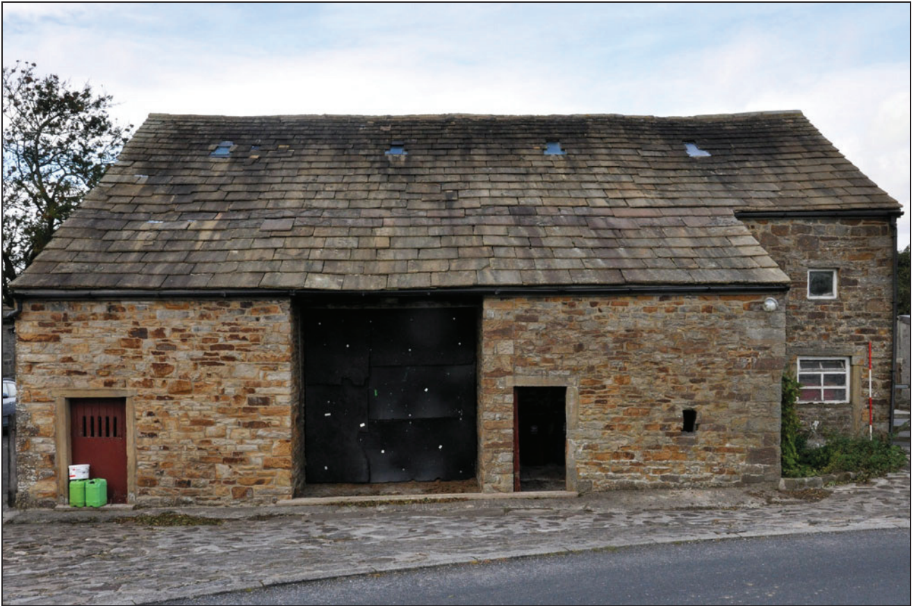
Photo 3: Front elevation of the barn
