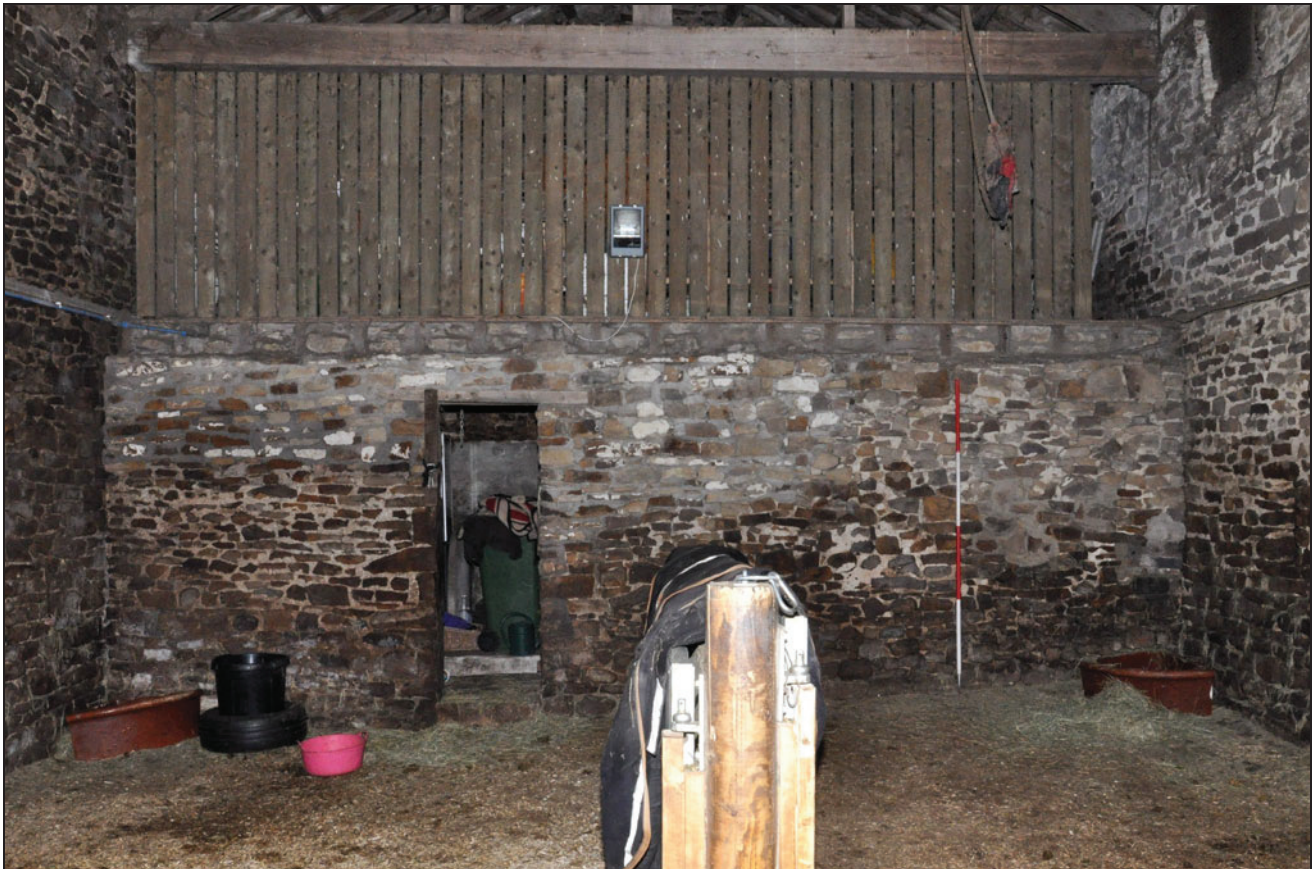
Photo 20: Cross-wall in barn, looking north-east
