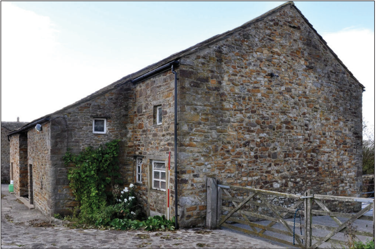
Photo 9: The barn, looking south-west
