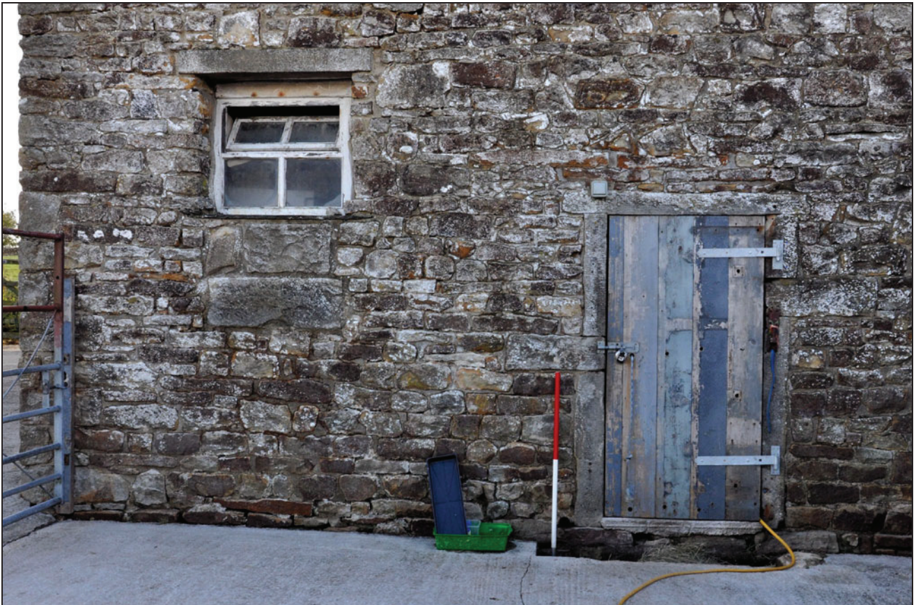
Photo 18: Detail of openings, north-east end of rear elevation
