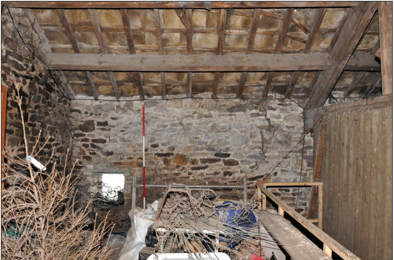
Photo 28: Loft over north-east shippon, looking south-east
