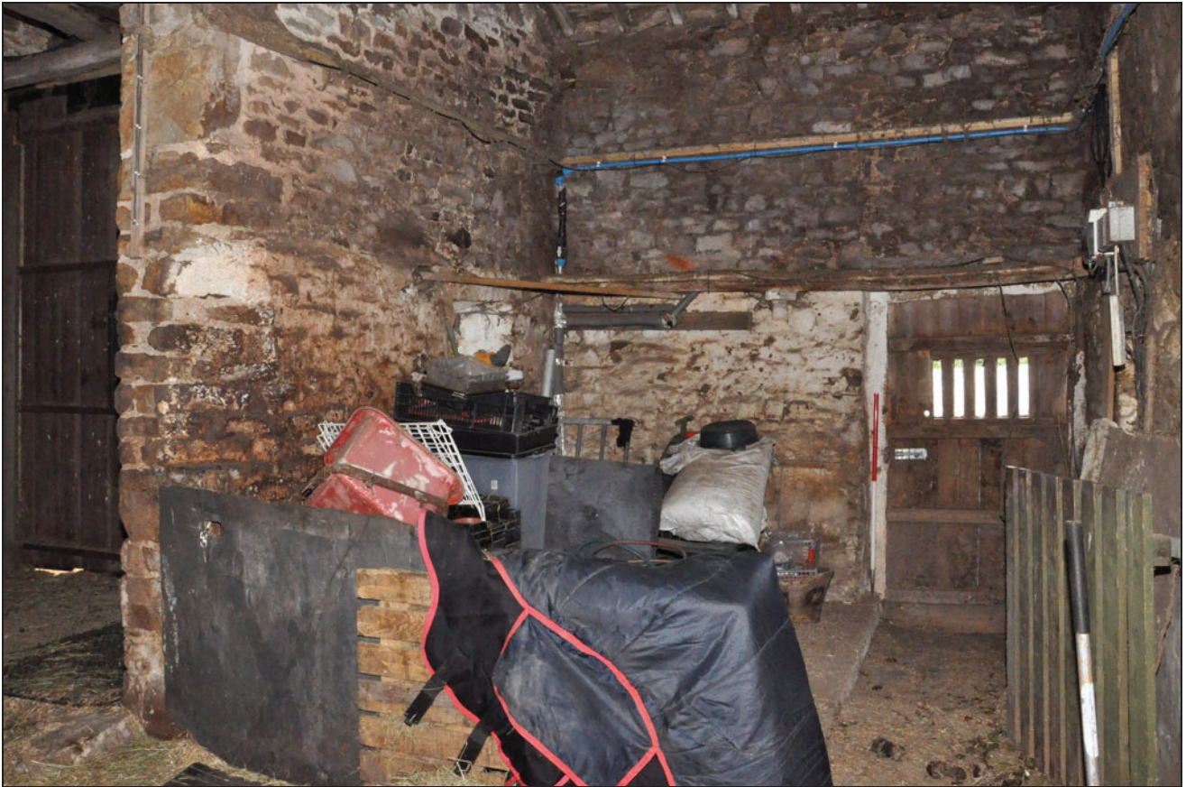
Photo 24: Former shippon, looking south-east, with slate uprights
