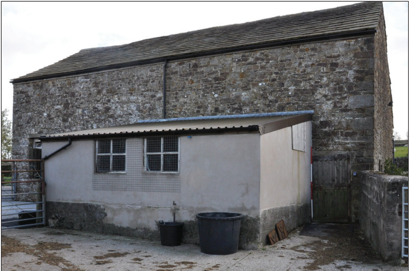
Photo 14: Rear of the barn, looking east, with modern lean-to in foreground
