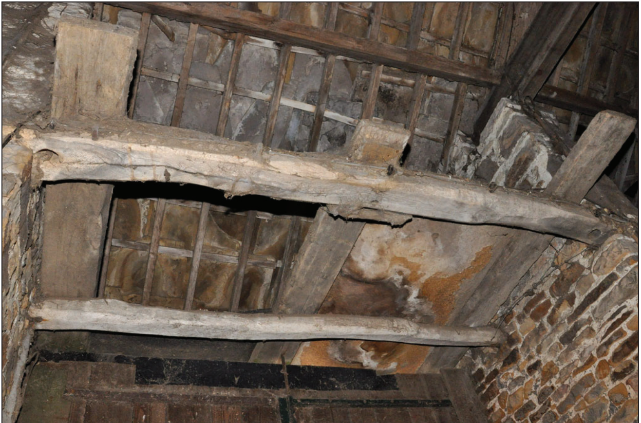
Photo 6: Detail of underside of doorway lintel, within porch
