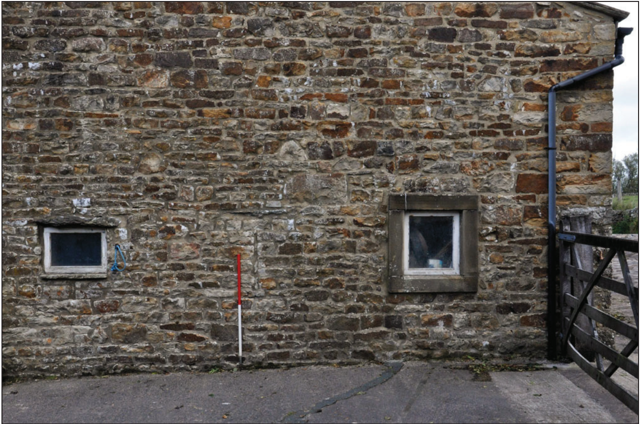
Photo 13: Detail of openings in south-west gable
