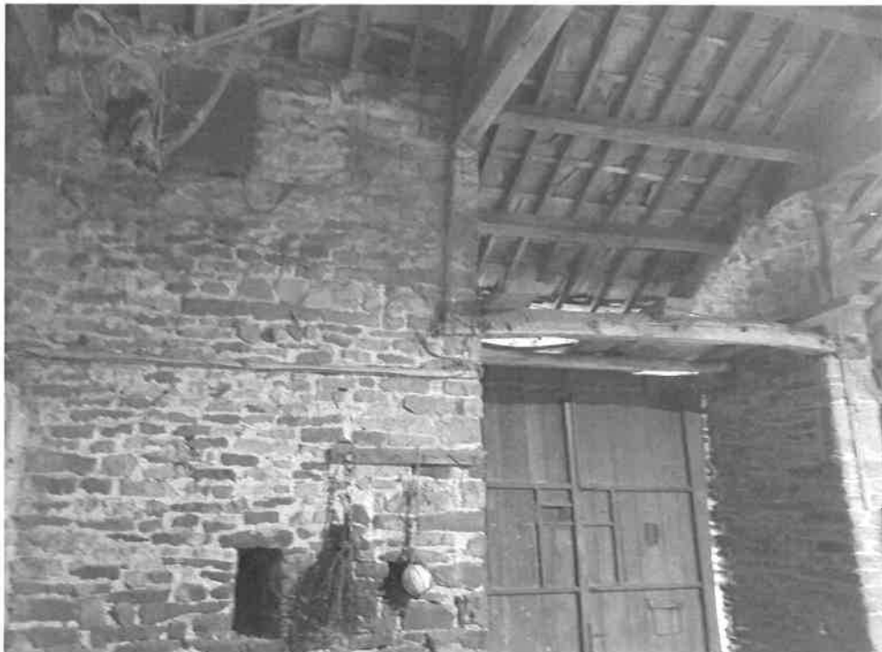
INTERNAL FRONT WALL
