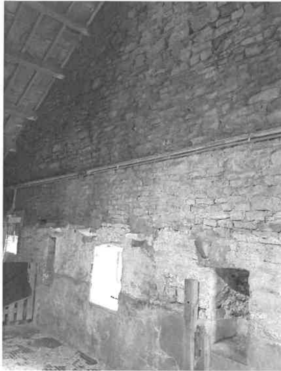
INTERNAL LEFT HAND WALL
