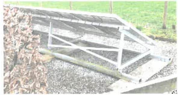
Existing photovoltaic panels have been relocated to a more efficient position
