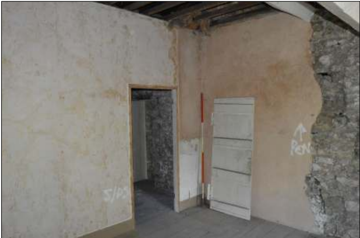
PL60: View north within first floor unit 06.
