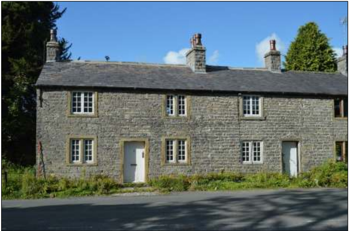
PL03: View of the south facing front elevation of the 5 / 7 Gisburn Road.
