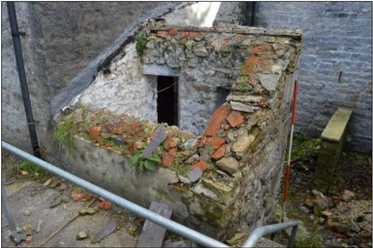
PL10: View of the rear of the outbuilding to the north side of the building.
