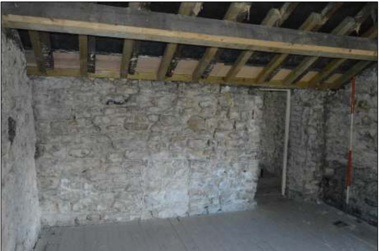
PL48: View south within first floor rear outshut unit 09. View also shows the reverse of the closed up former window opening.
