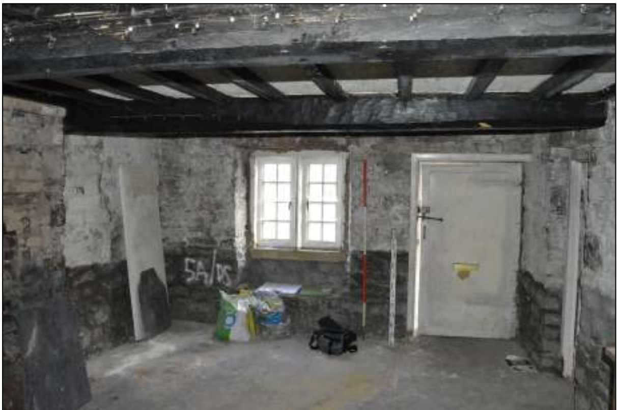
PL18: View south within ground floor unit 02.
