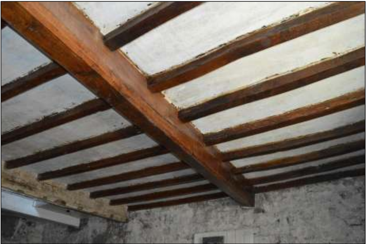
PL33: Timber floor structure and ceiling over ground floor unit 03.
