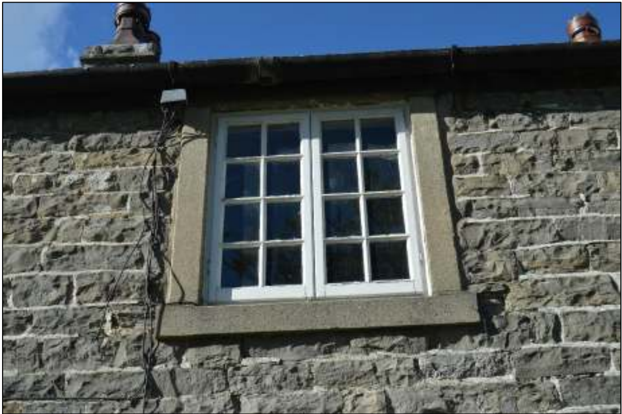
PL08: Concrete jambs, head and cill noted to the first-floor window to No. 7 Gisburn Road.
