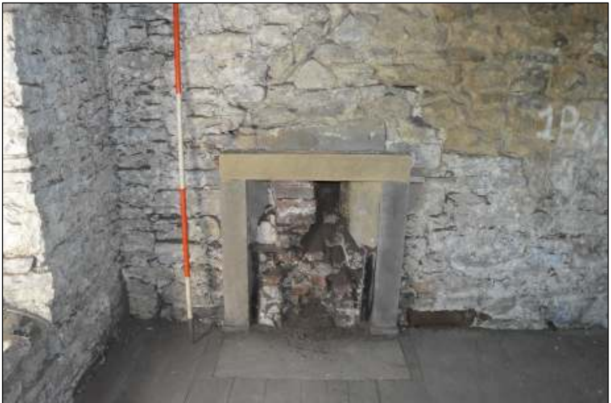
PL41: Fireplace located to first floor unit 08.
