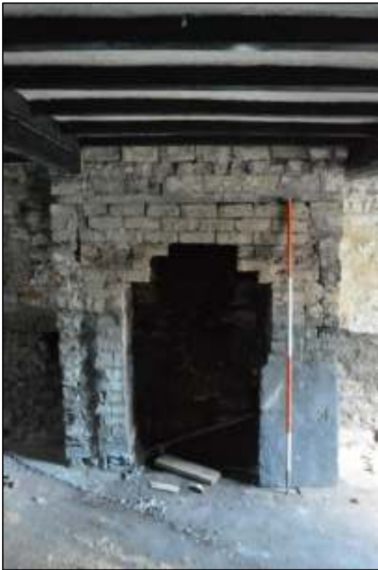
PL19: (Left) view of existing fireplace and chimney breast in ground floor unit 02. P20 (Right) Blocked up opening between ground floor unit 02 and 01.
