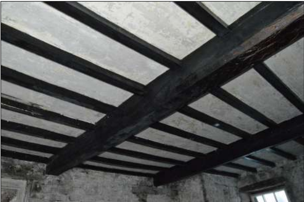
PL21: Timber floor structure and ceiling over ground floor unit 02.
