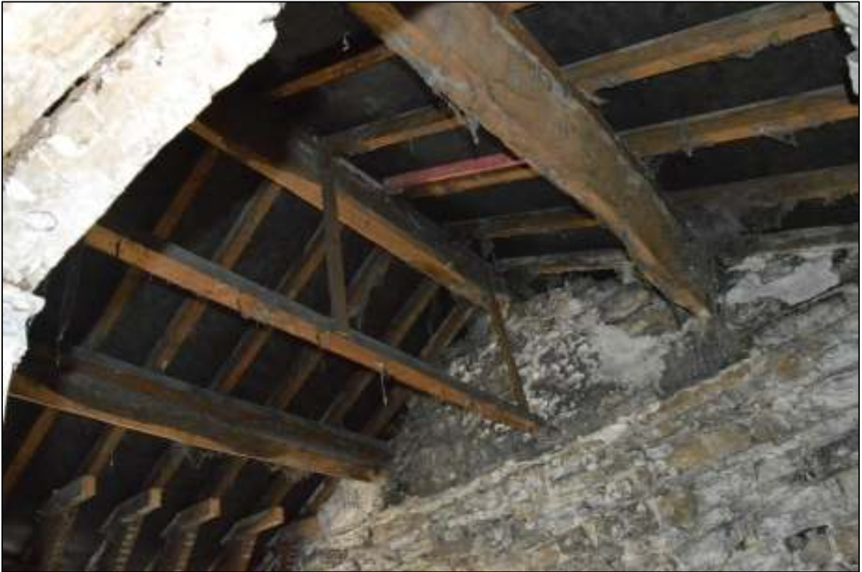
PL58: View of roof structure over first floor unit 05 (ceiling removed).
