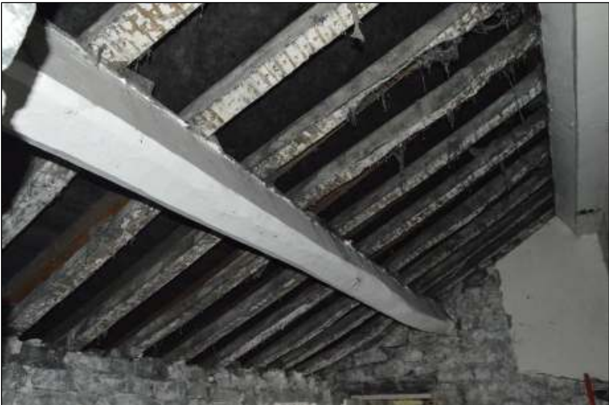
PL55: View of first floor roof structure over the first-floor unit 07.
