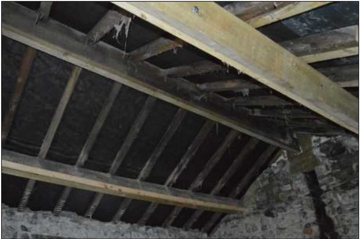
PL51: View of repaired timber roof structure to the north roof pitch above first floor rear outshut unit 09.
