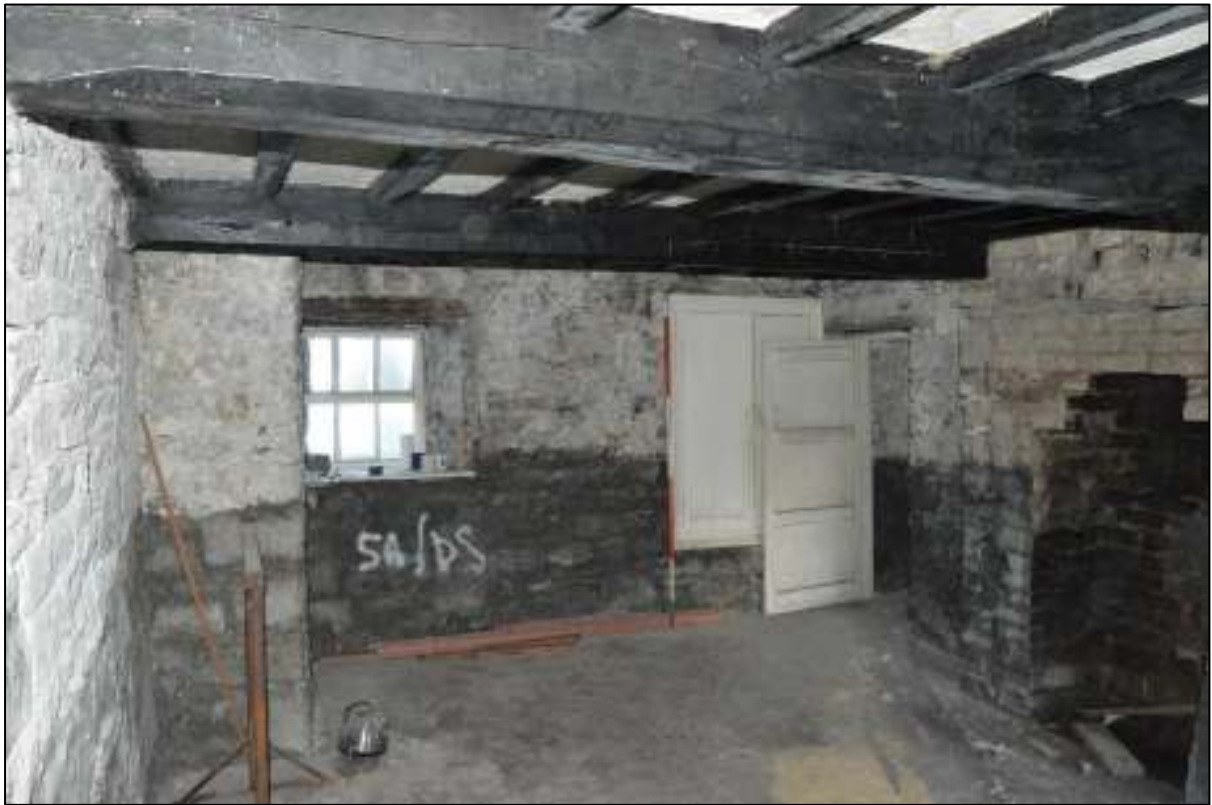
PL18: View north within ground floor unit 02.
