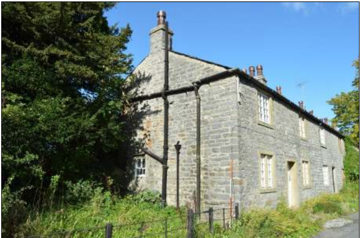
PL04: View of the east facing elevation of 5 / 7 Gisburn Road.
