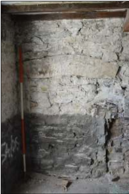
PL30 (Left) former closed up opening / recess to the west wall of ground floor unit 03. PL31 (Right) Fireplace present to ground floor unit 03.
