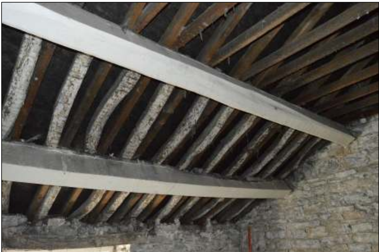
PL61: View of roof structure over first floor unit 06.
