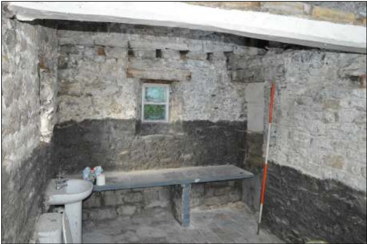
PL22: View north within ground floor unit 01.
