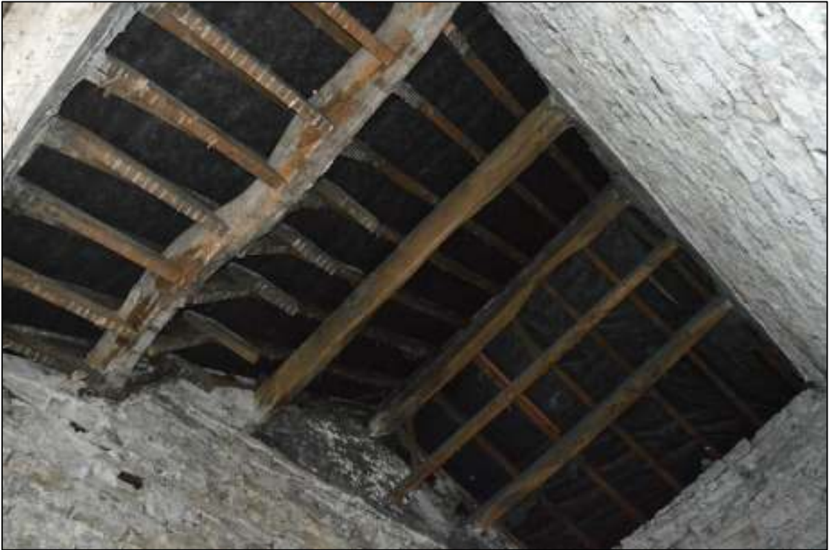
PL26: View of timber roof structure over ground floor unit 01 / first floor unit 05)
