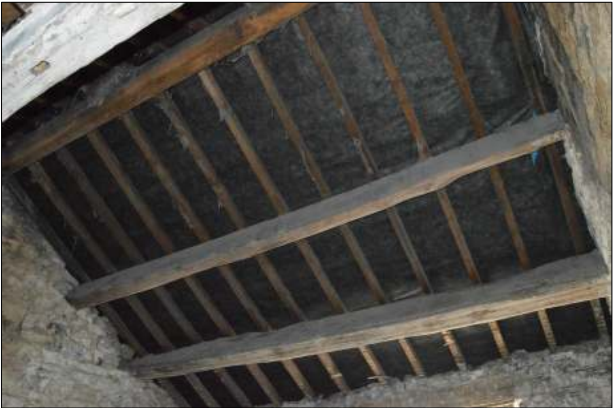
PL44: View of the south roof pitch over first floor unit 08.
