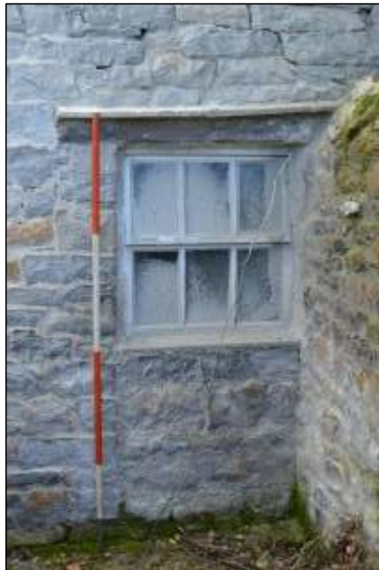
PL17: Closed up former door opening (now window) to the rear north elevation.
