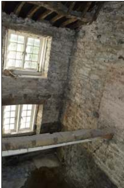
PL57: View of ground floor unit 01 and unit 05 (floor removed).
