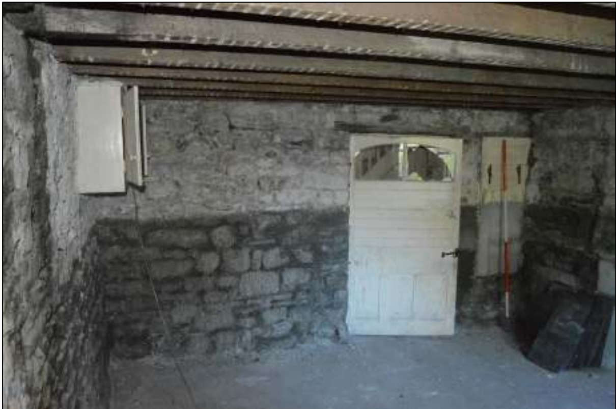
PL35: View south within the ground floor rear outshut unit 04.
