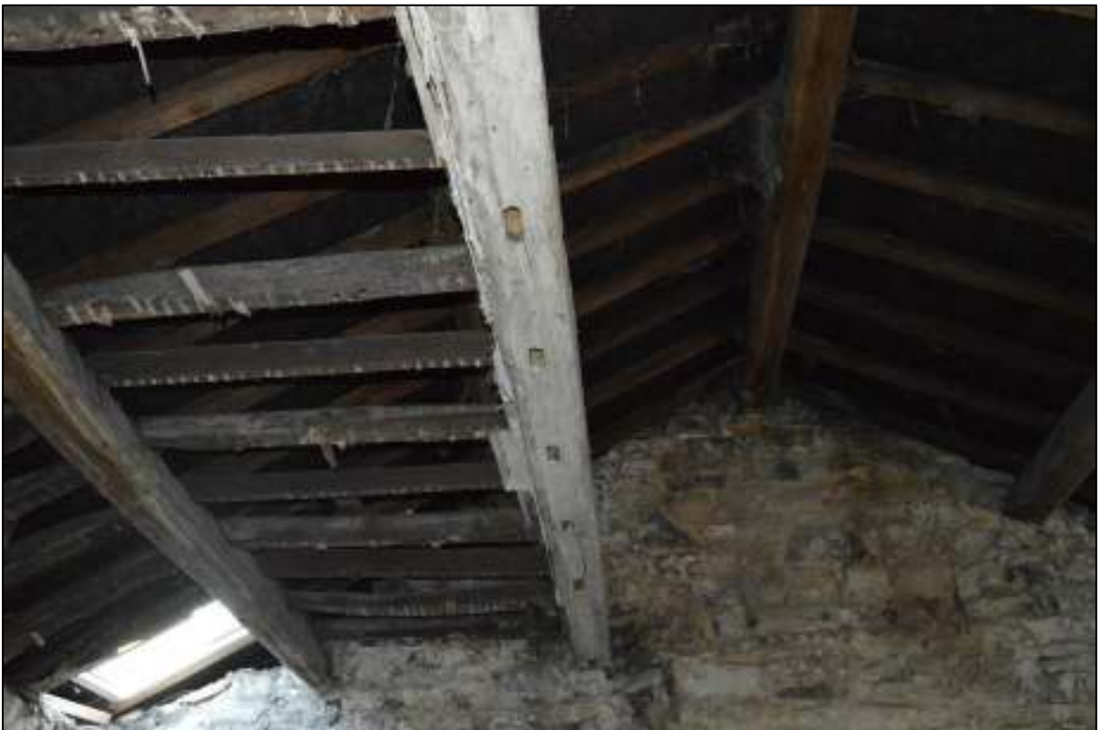
PL45: View of timber beam to the rear of first floor unit 08 with possible stave holes for former wattle and daub wall.
