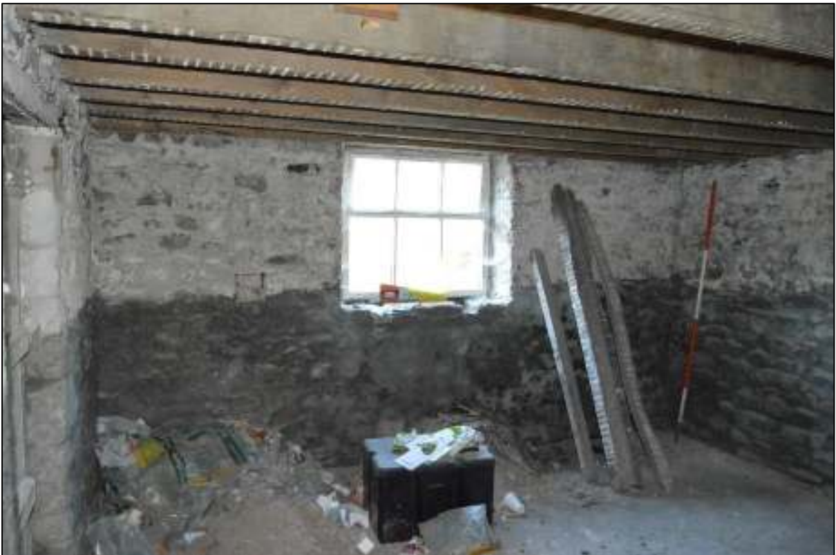
PL34: View north within the ground floor rear outshut unit 04.
