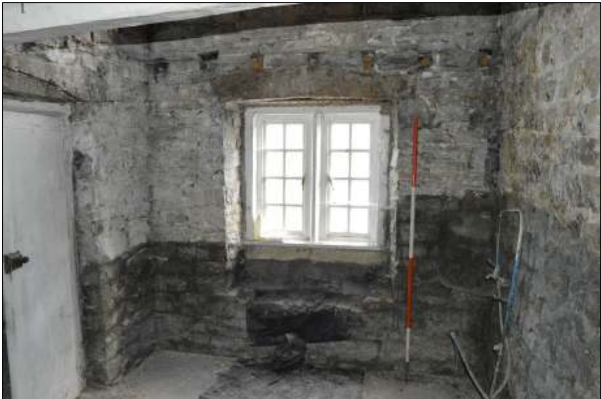
PL23: View south within ground floor unit 01.
