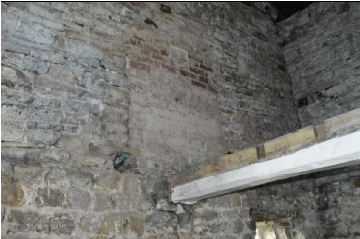
PL25: View of closed up fireplace located at first floor unit 05 (viewed from ground floor level)
