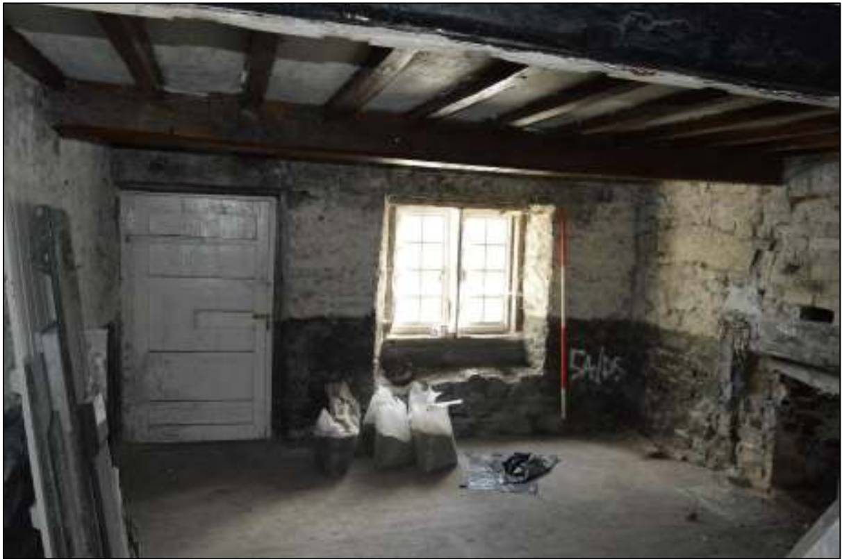
PL28: View south within ground floor unit 03.
