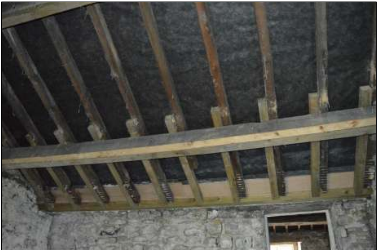
PL50: View of repaired timber roof structure to the south roof pitch above first floor rear outshut unit 09.
