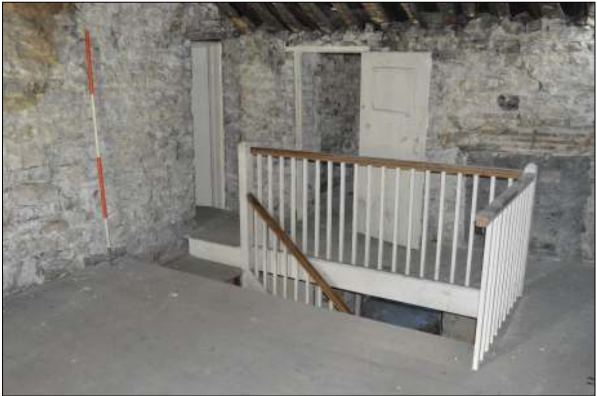
PL40: View north within first floor unit 08.
