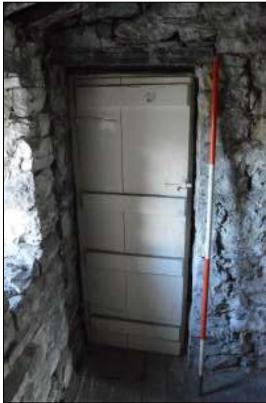
PL56: View of plank and batten door located between first floor unit 07 and 08.
