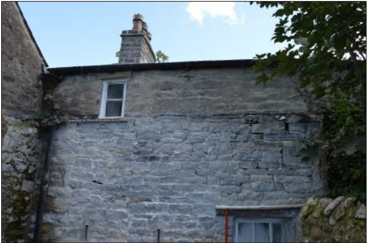
PL16: View of the first floor of the rear north facing elevation.
