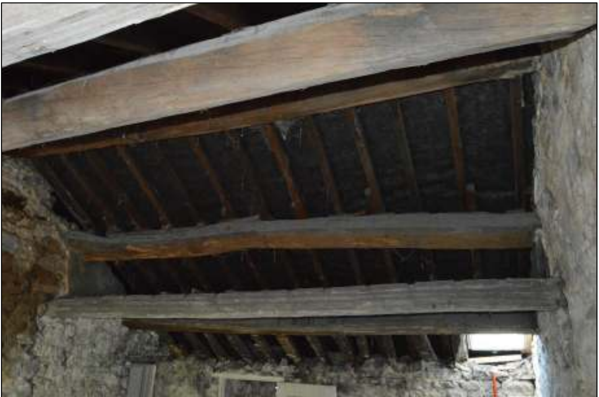
PL43: View of the north roof pitch over first floor unit 08.
