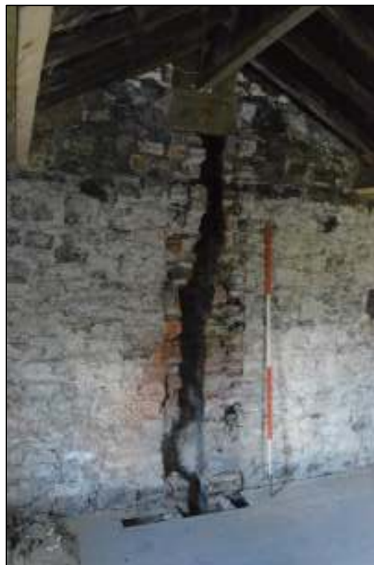
PL52: Former flue void to the east wall within first floor rear outshut unit 09.
