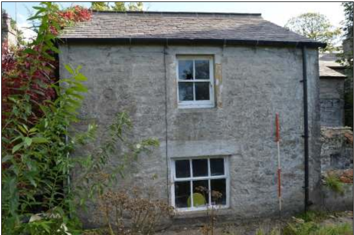
PL09: View of the north facing elevation of the rear outshot.
