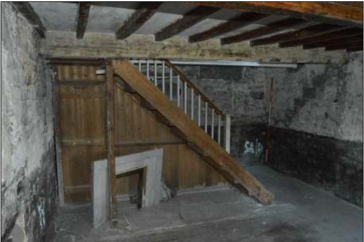
PL27: View north within ground floor unit 03
