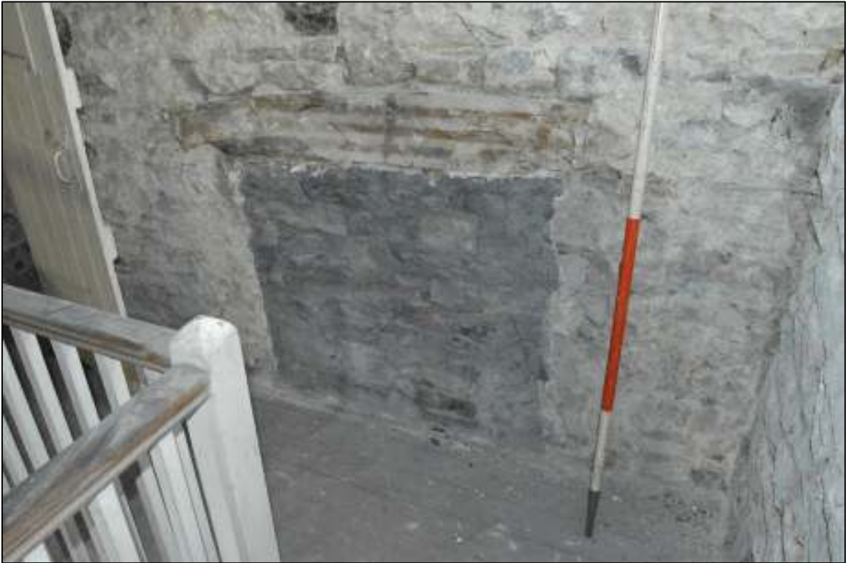
PL42: Closed up former window located to the former historic staircase location to the north east corner of first floor unit 08.
