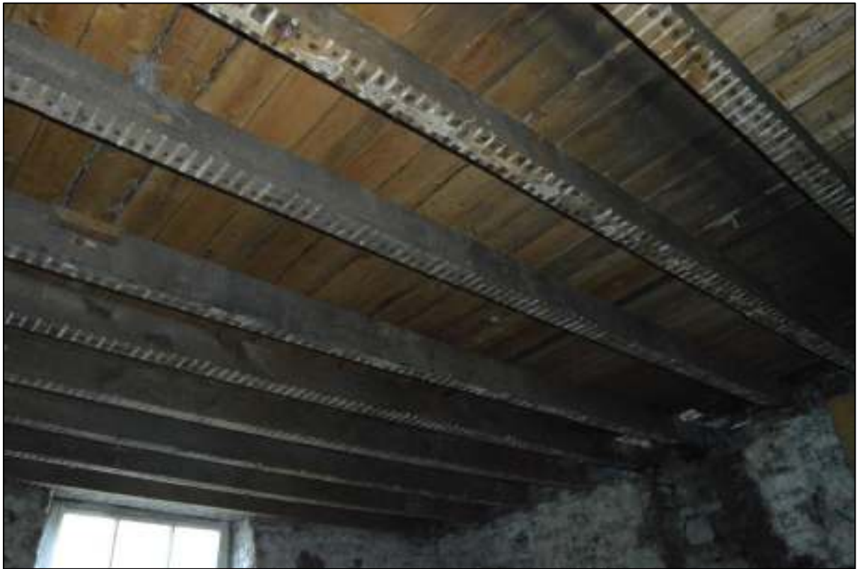
PL38: Timber floor structure over ground floor rear outshut unit 04.
