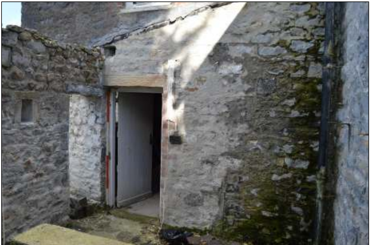
PL13: View of the ground floor level east elevation of the rear outshut.
