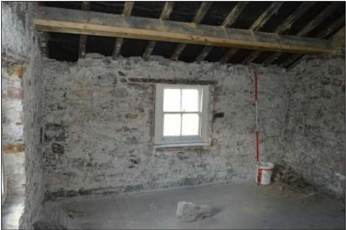
PL49: View north within first floor rear outshut unit 09.
