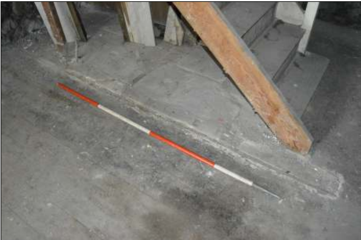
PL32: Location of removed wall and visible remnants of stone flag floor to the staircase location in ground floor unit 03.
