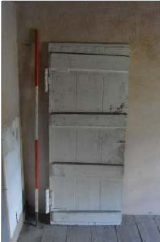
PL62: View of plank and batten door placed within first floor unit 06.
