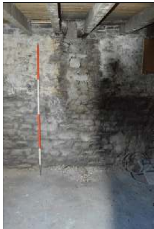
PL36: (Left) Closed up former opening to the east wall and former closed up opening (now cupboard) to the south wall to ground floor rear outshut unit 04. PL37 (Right) former chimney breast location to ground floor rear outshut unit 04.
