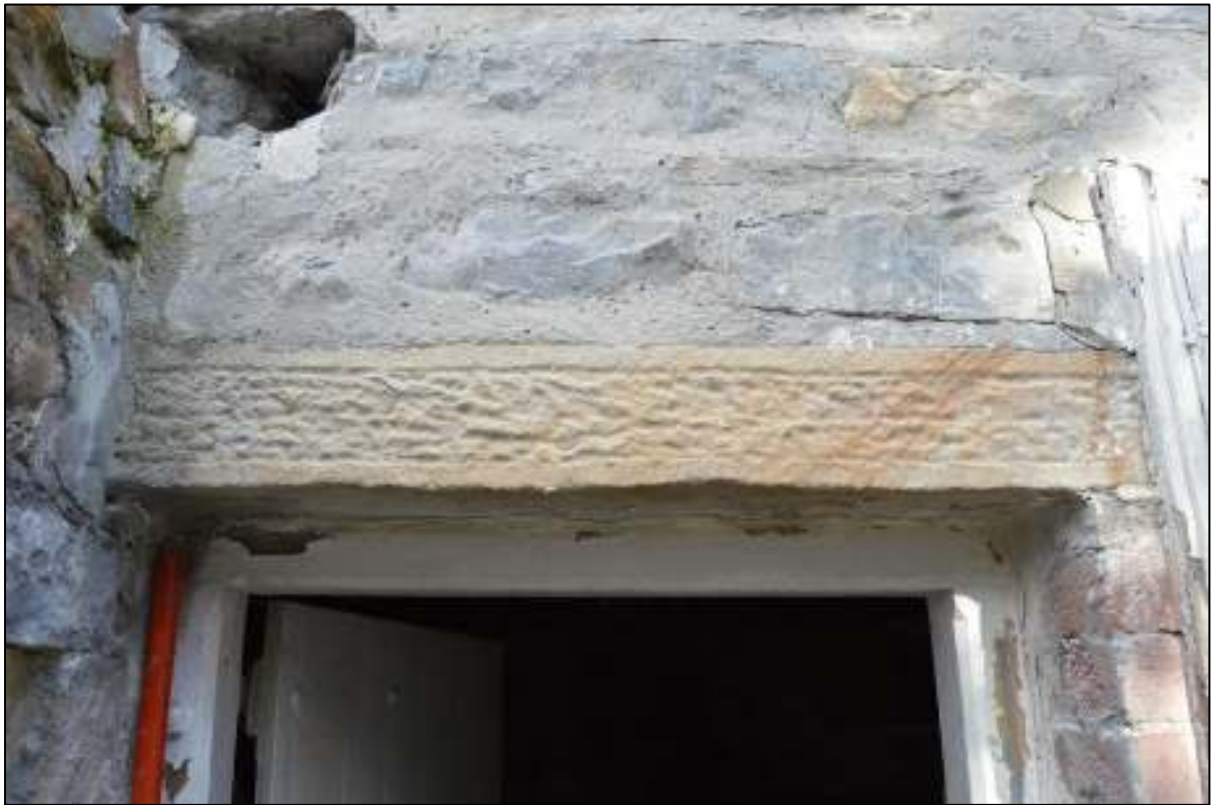
PL14: View of the rusticated stone head over the outshut door to the east elevation.
