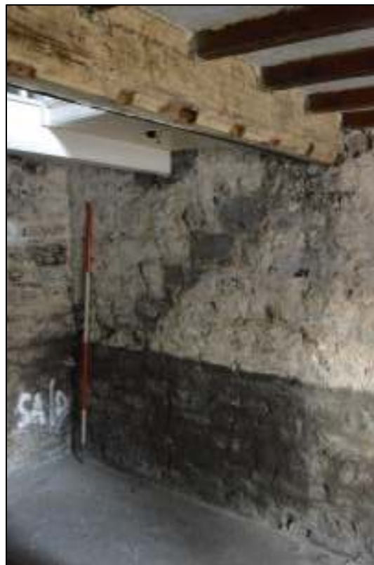
PL29: Location of former historic staircase.
