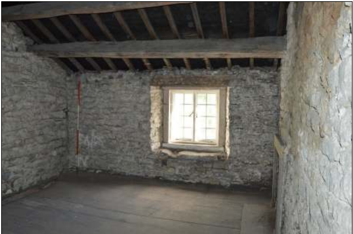
PL39: View north within first floor unit 08.
