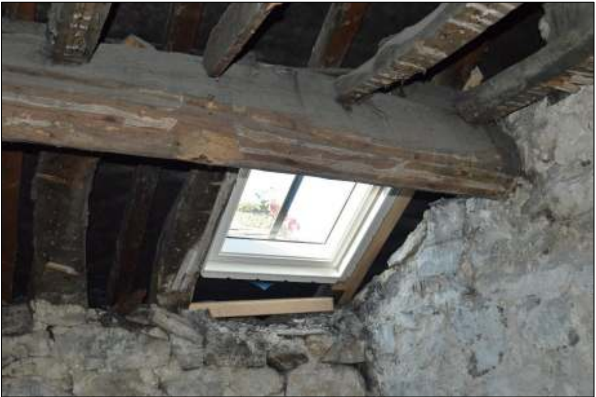
PL46: Inserted roof light to the north east corner of first floor unit 08.
