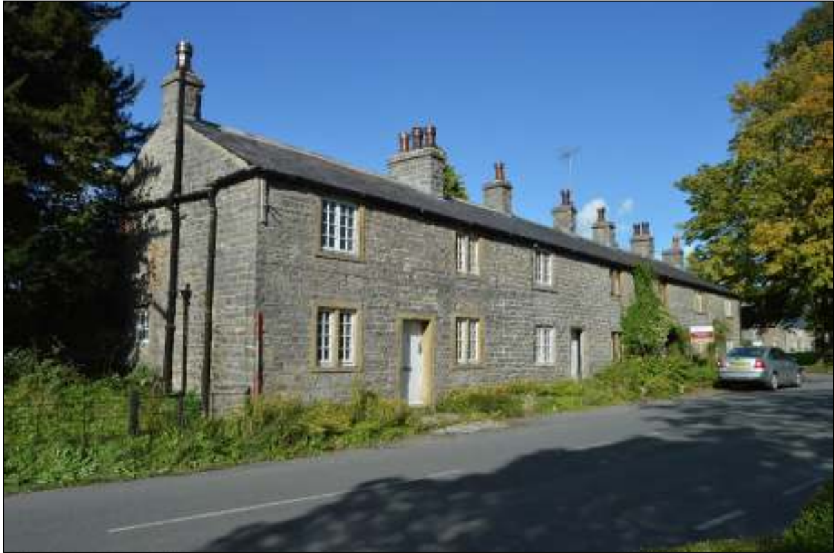
PL02: View of 5 / 7 Gisburn Road from the south west.
