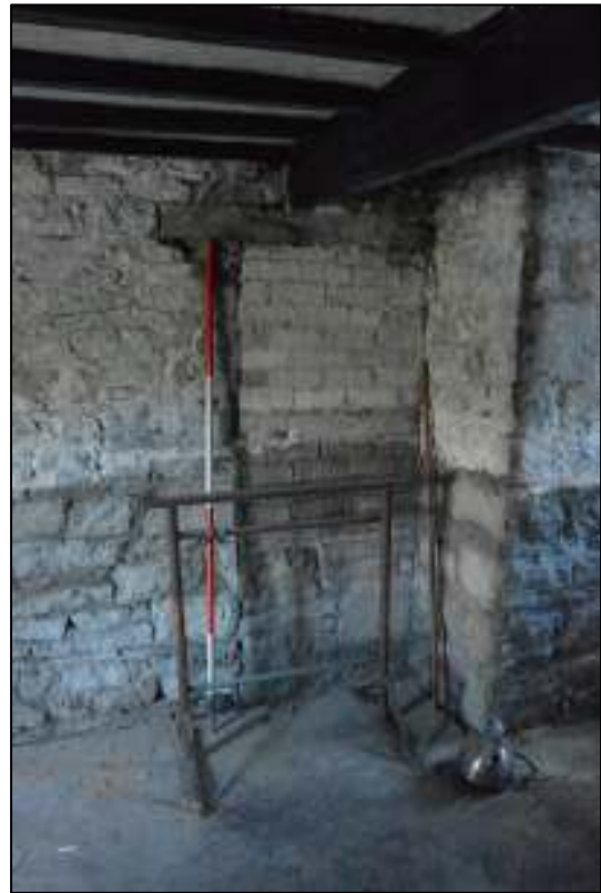
PL19: (Left) view of existing fireplace and chimney breast in ground floor unit 02. P20 (Right) Blocked up opening between ground floor unit 02 and 01.
