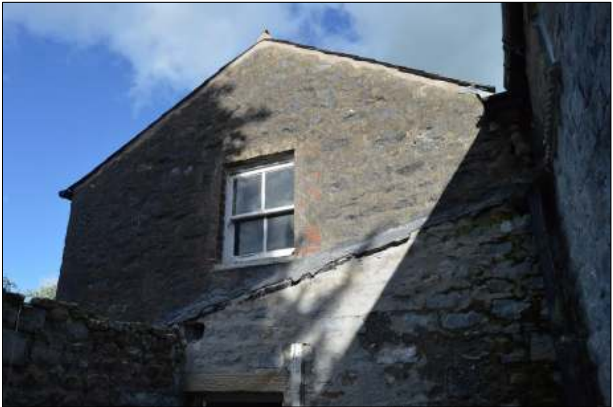
PL12: View of the first-floor level east elevation of the rear outshut.
