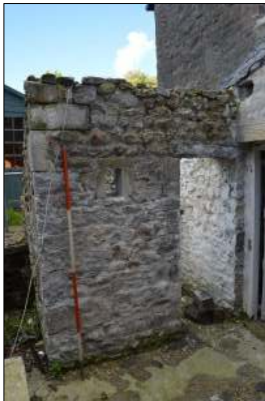
PL11: View of the front of the rear outbuilding.
