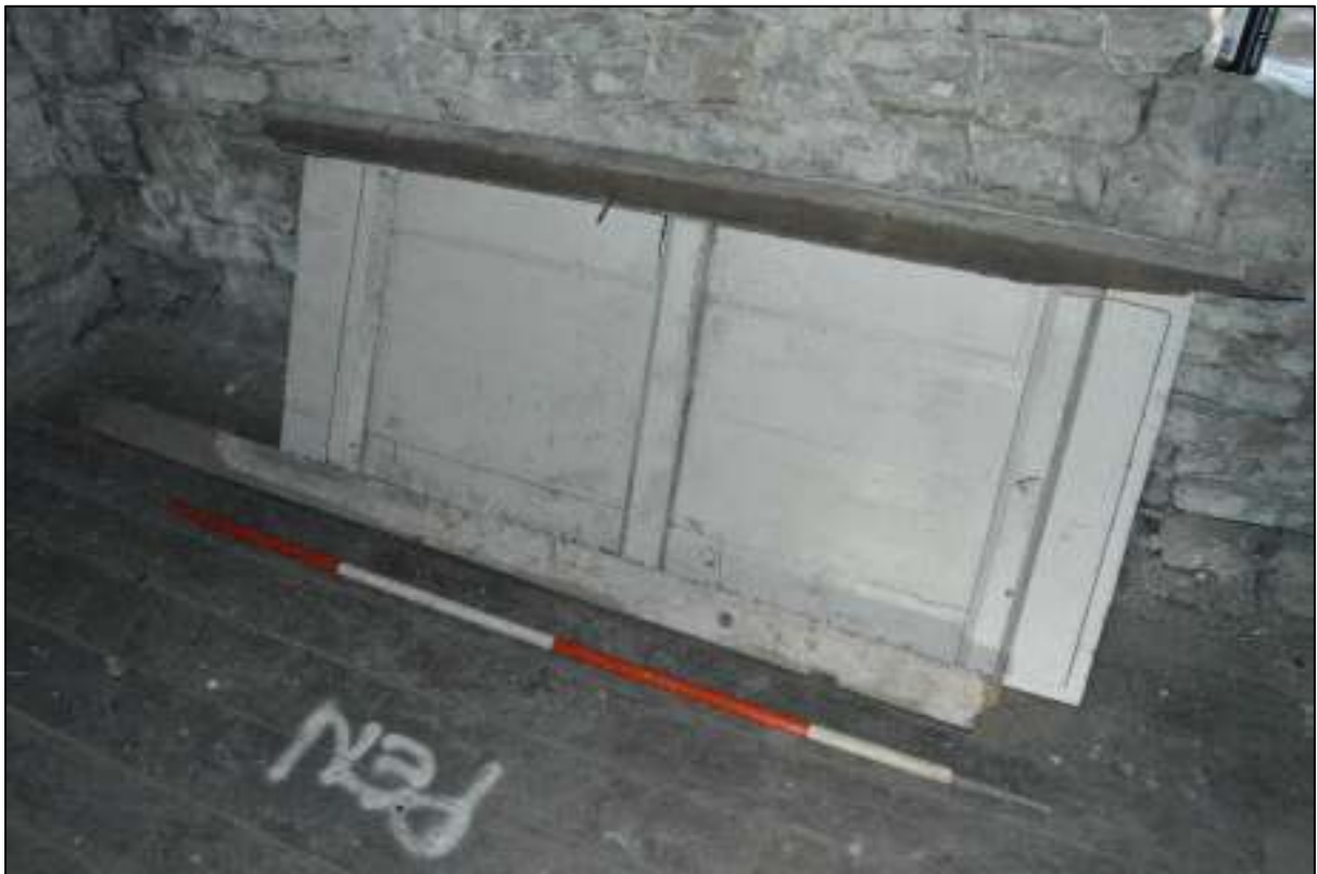
PL63: View of plank and batten door placed within first floor unit 07.
