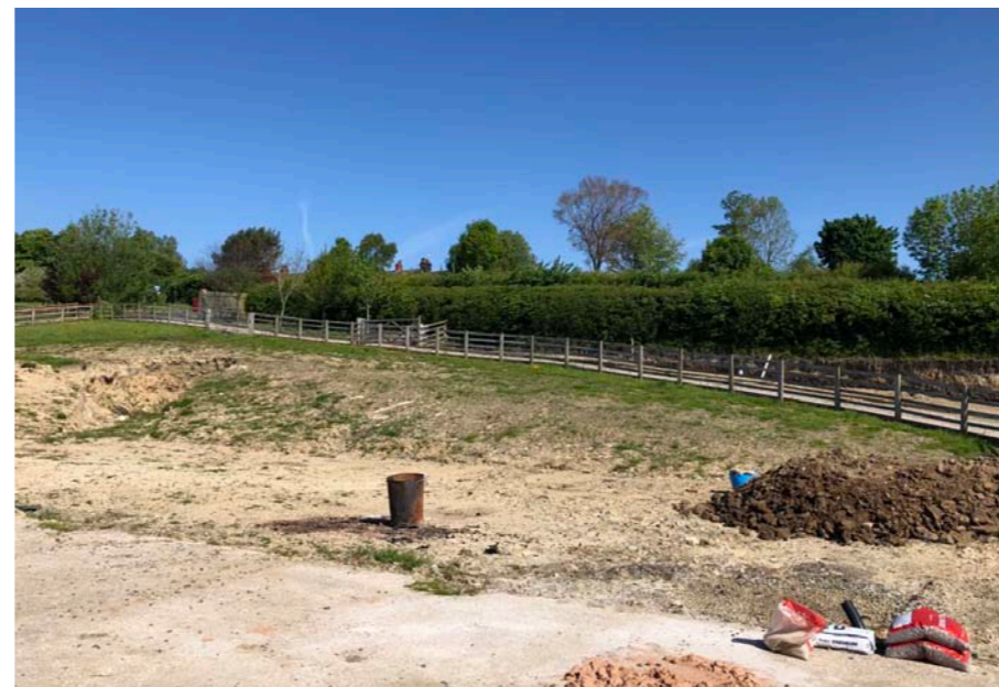
View of private access road to the North of the site.
