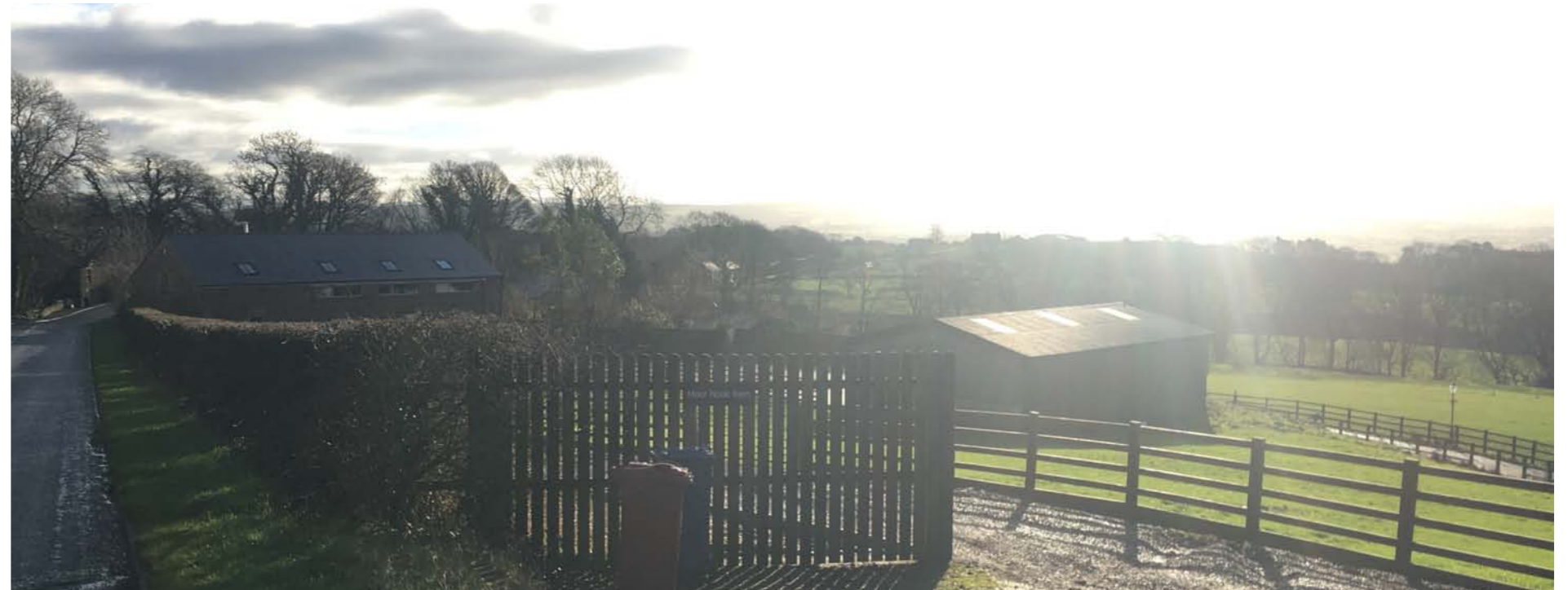
View of Moor Nook Barn, taken from the North West on Clitheroe Road
