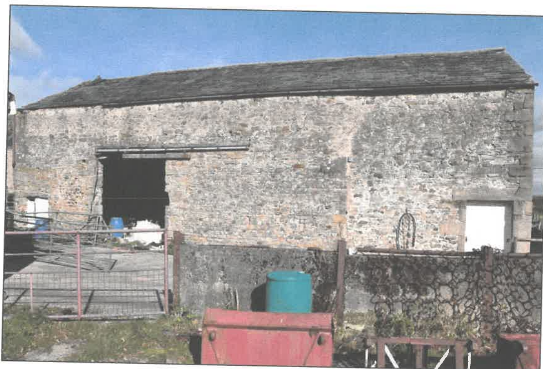
Photo 10 Barn: south front
