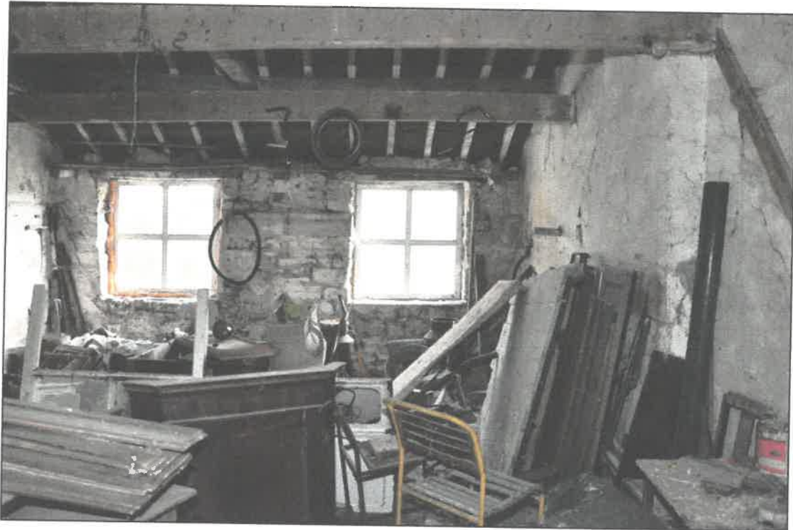
Photo 9 Garage/trap house: first floor, latterly joiner's workshop
