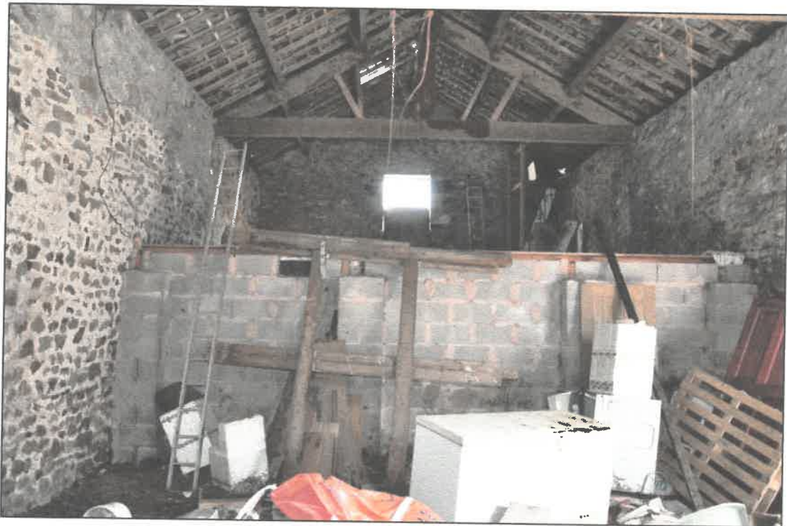
Photo 13 Barn: blockwork enclosing ice-creamery, east end
