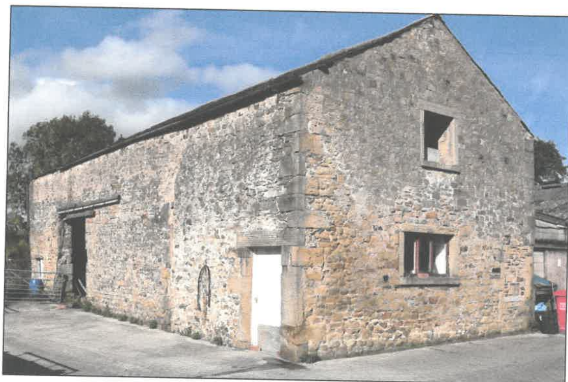
Photo 11 Barn: 19th century addition, east end
