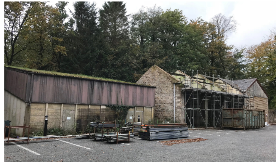
Fig 5. Photographs of the building as existing
