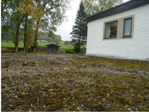
The Garage flat roof
