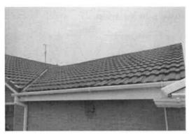
The roof has loft space present. A modern breathable membrane suggests some recent re-roofing work as part of the addition of the extension.
