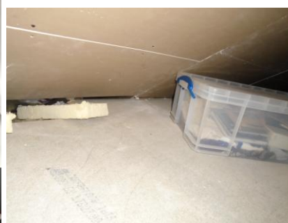
Main roof void
