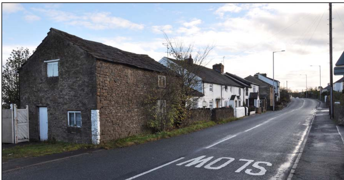
Photo 1: The outbuilding (left), looking east up Ribchester Road
