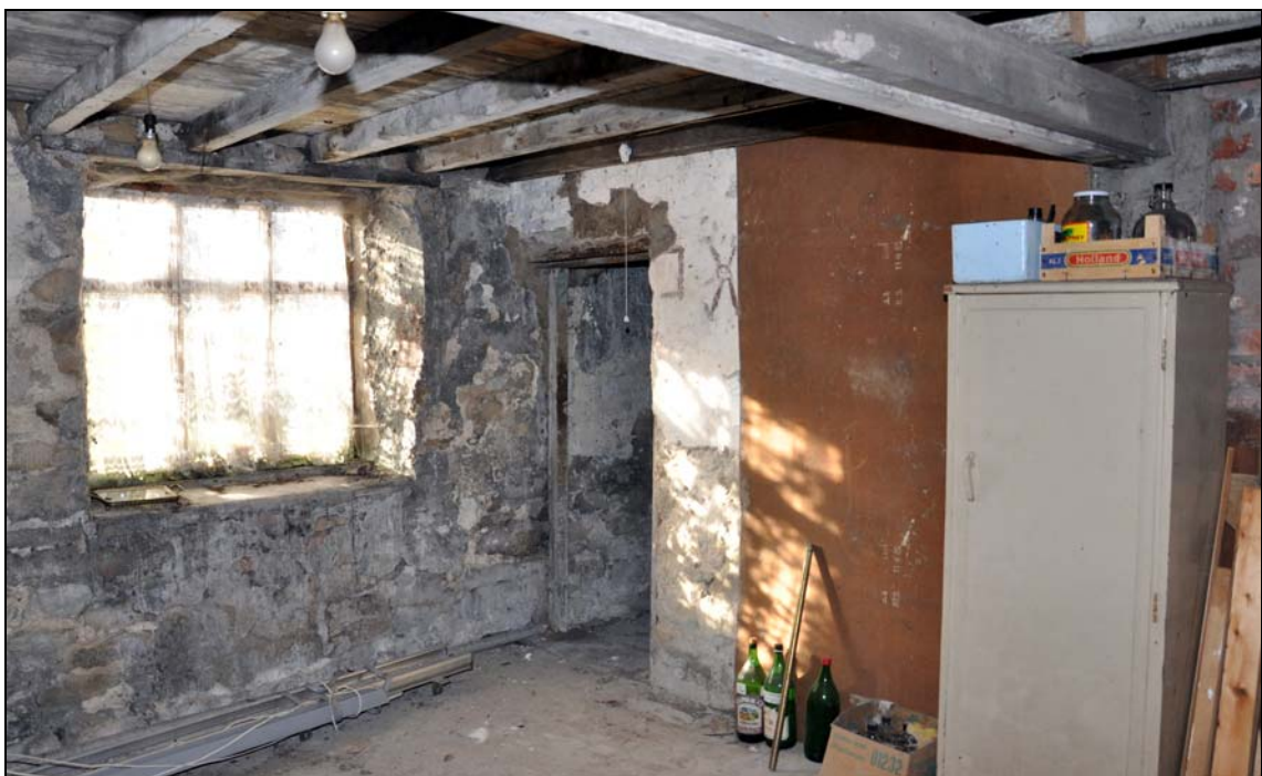
Photo 4: Ground floor (east room)
