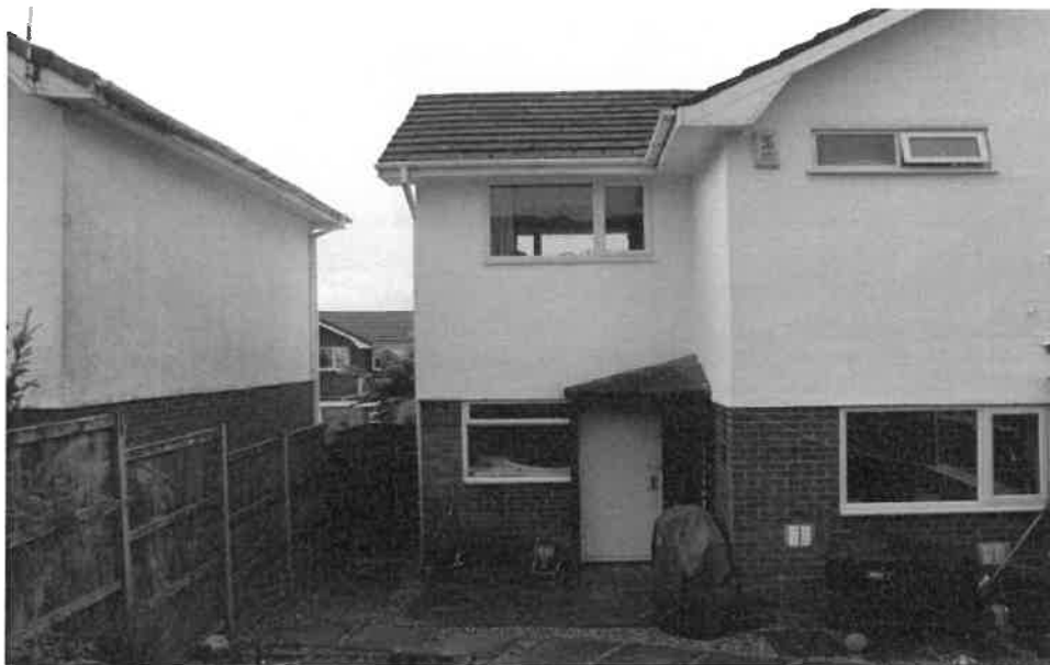
Part existing Rear Elevation, northern facing
