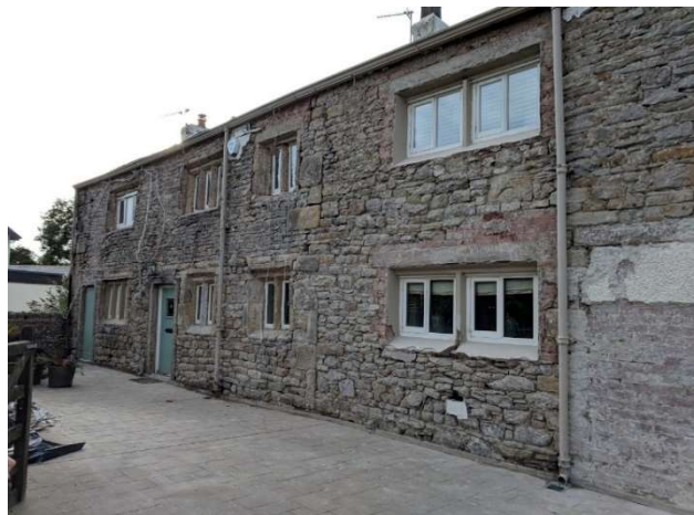
Figure 1 – Front Elevation with the render removed
