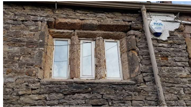
Figure 2 – Photo showing damaged stone mullion
