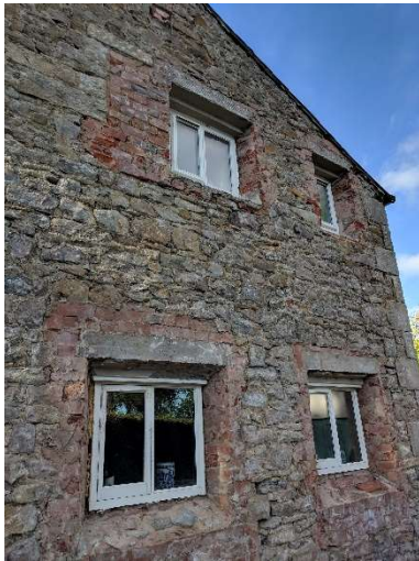
Figure 3 – Photo showing inappropriate/non-original materials to end elevation
