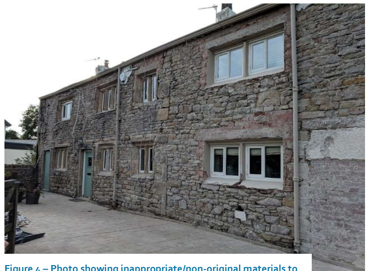
Figure 4 – Photo showing inappropriate/non-original materials to front elevation
