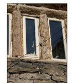
Where the stone cill and mullion is damaged, cut the stone removing rough edges. Then create templates of the cut sandstone and shape new stone to match. New matched stone pieces are then to be fixed in place using the previously agreed lime
