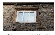
Provide temporary support to the existing opening and remove existing window. Install new sandstone stone mullions to match the existing first floor mullions. Where the stone cill is damaged, cut the stone removing rough edges. Then create template of the cut sandstone and shape new stone to match. New matched stone to be fixed in place using the previously agreed lime mortar mix. Install new windows to match the existing windows in the property.
