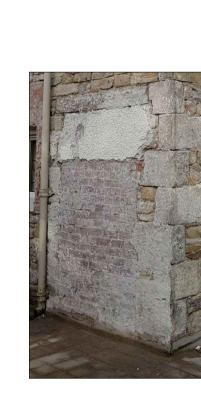
Removed existing brick and dispose of offsite. Make good the door jambs using reclaimed stone matching in colour and size. Create new hardwood timber door casing and hardwood door to match door 1. Fix in place and paint to match the existing.
