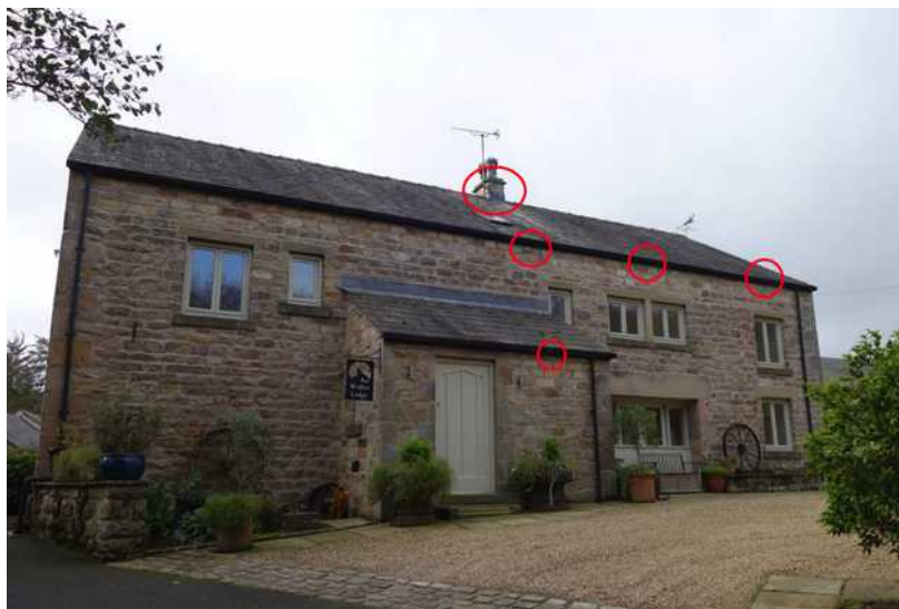
Bat roost locations identified during surveys on frontage (North) of property.
