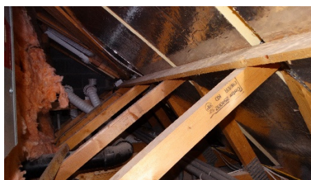
Figure 8: Rear eaves void
