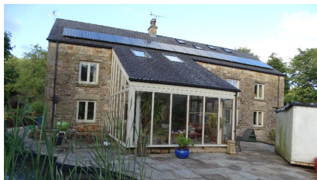
Figure 2: Rear (west) elevation
