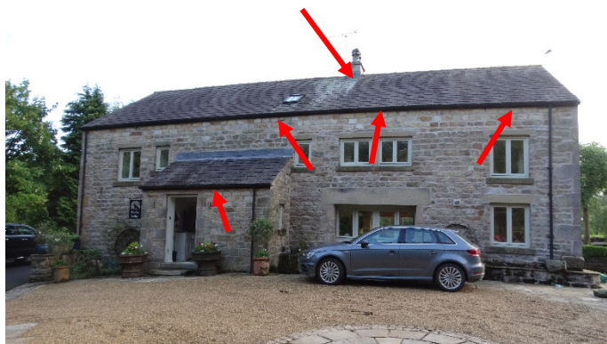
Figure 1: Front (east) elevation
