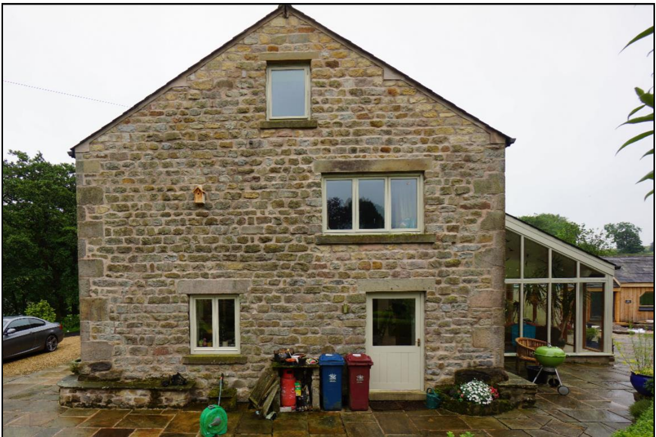
Figure 6) Northern elevation with inserted openings and raised gable
