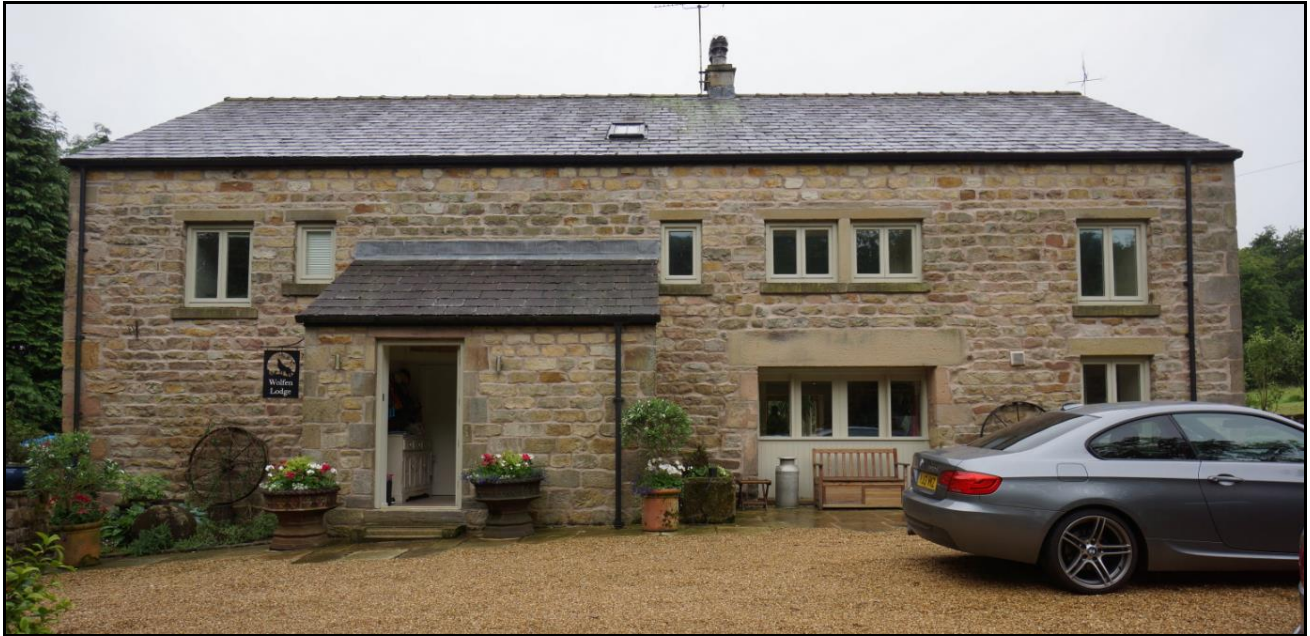
Figure 5) Eastern elevation with porch extension, inserted windows, reduced former cart entry and raised upper wall level above first floor lintels.
