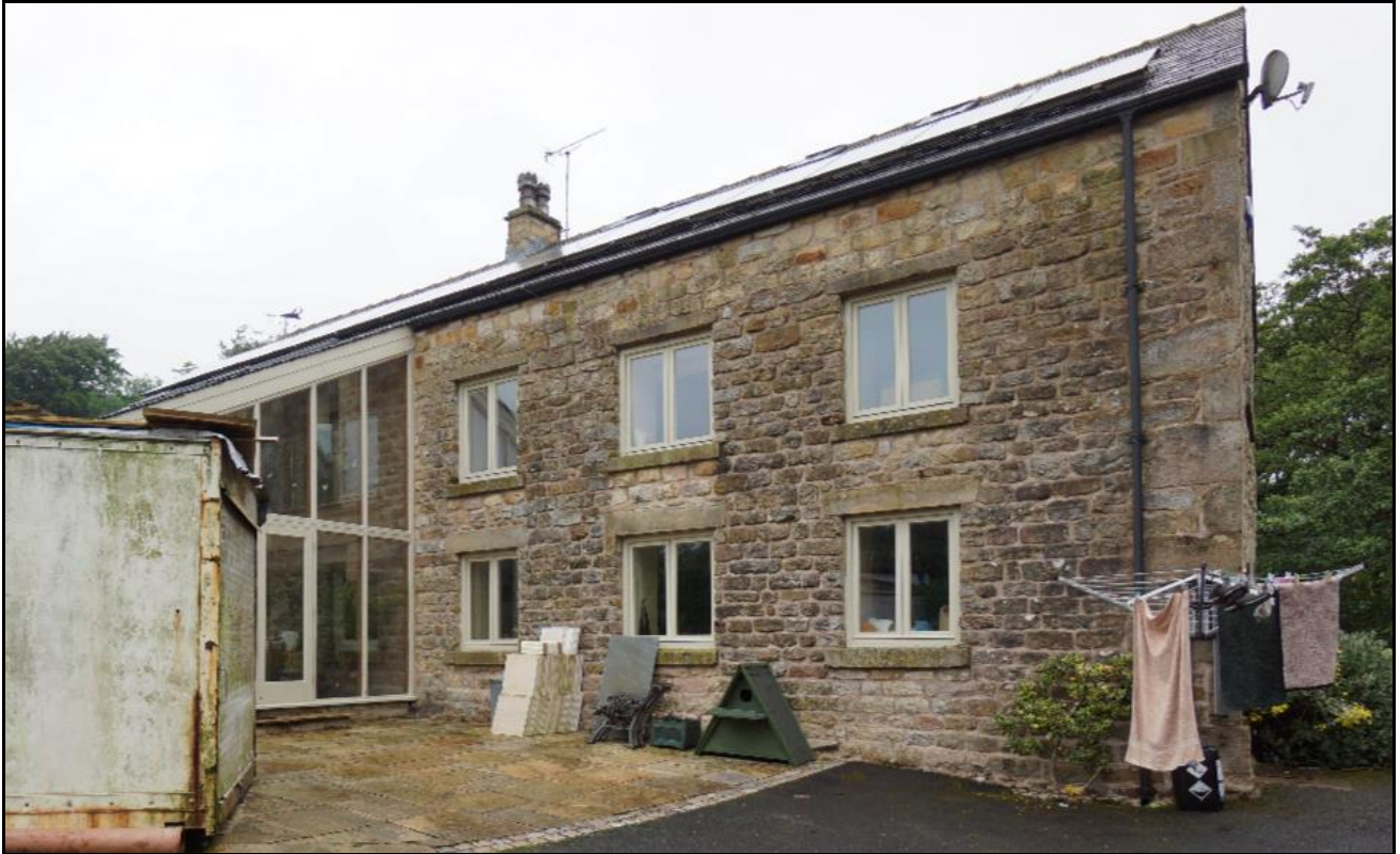
Figure 7) Western elevation wirth inserted windows and conservtory extension
