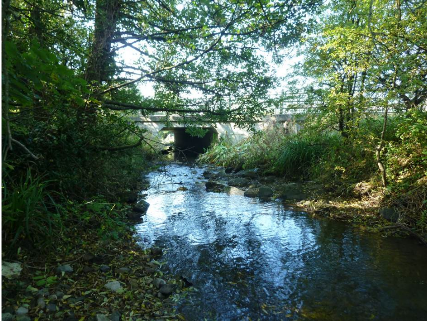
Photograph 7: Mearley Brook looking downstream towards Lincoln Way bridge.
