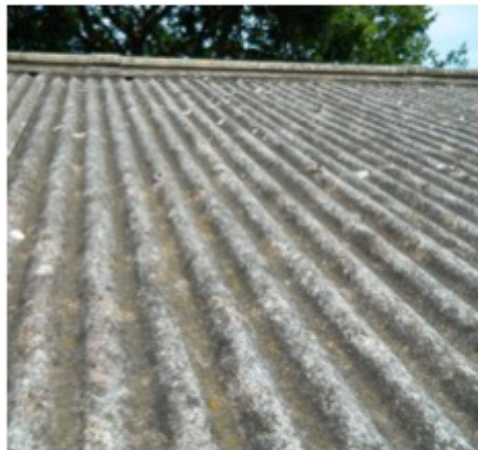
Fibre cement sheeting showing lichens, liverwort and moss growth
