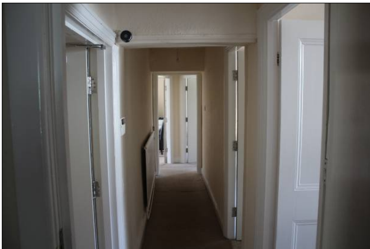
11. The first floor corridor leading from the staircase dates from this time
