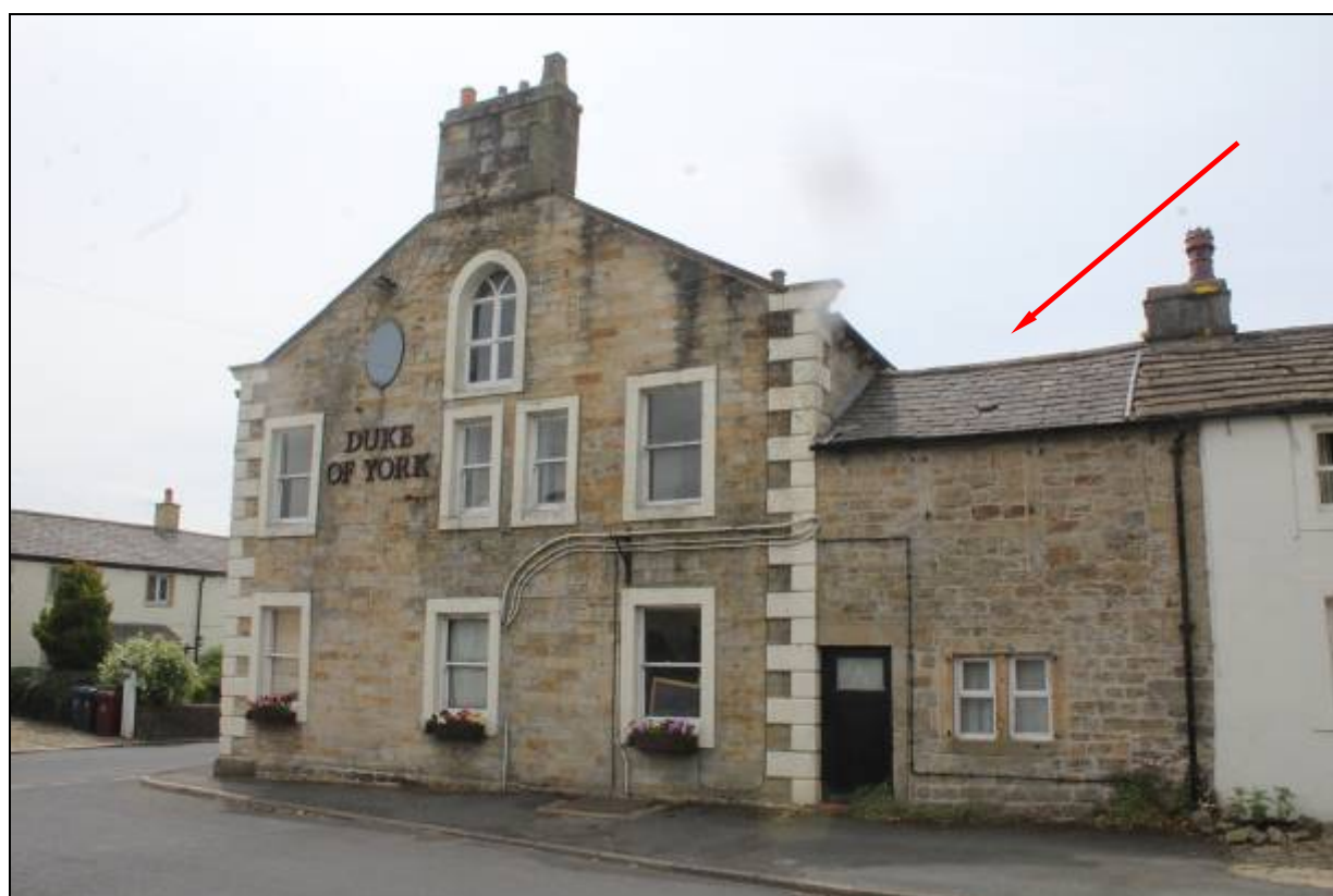
7. Low rear element to Main Street appears to have been part of a stabling range
