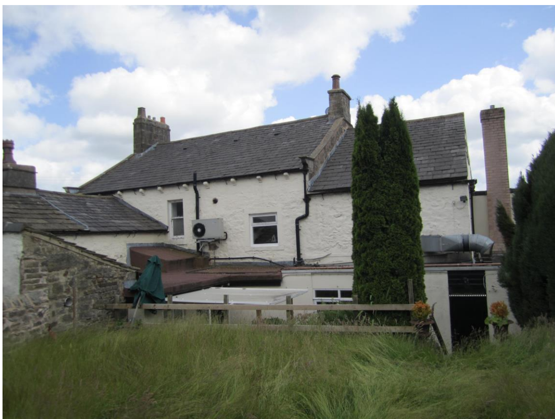
Single storey rear extension to be demolished
