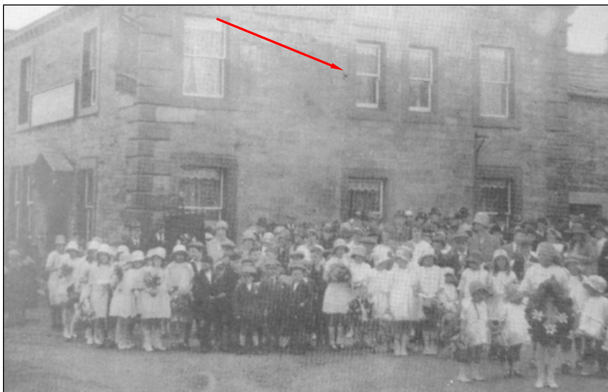
6. By circa 1926, the date of this photograph, two new first floor windows had been inserted, following repositioning of the staircase
