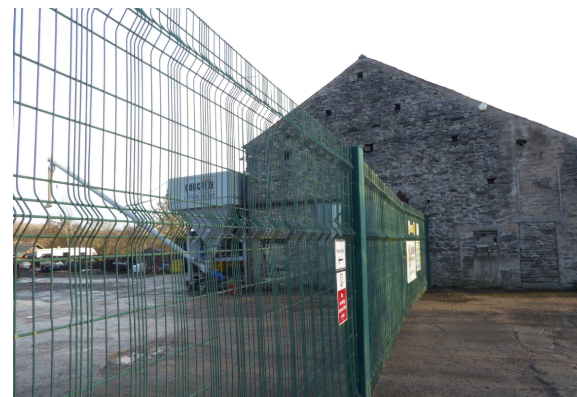
Security Fence and Gate
