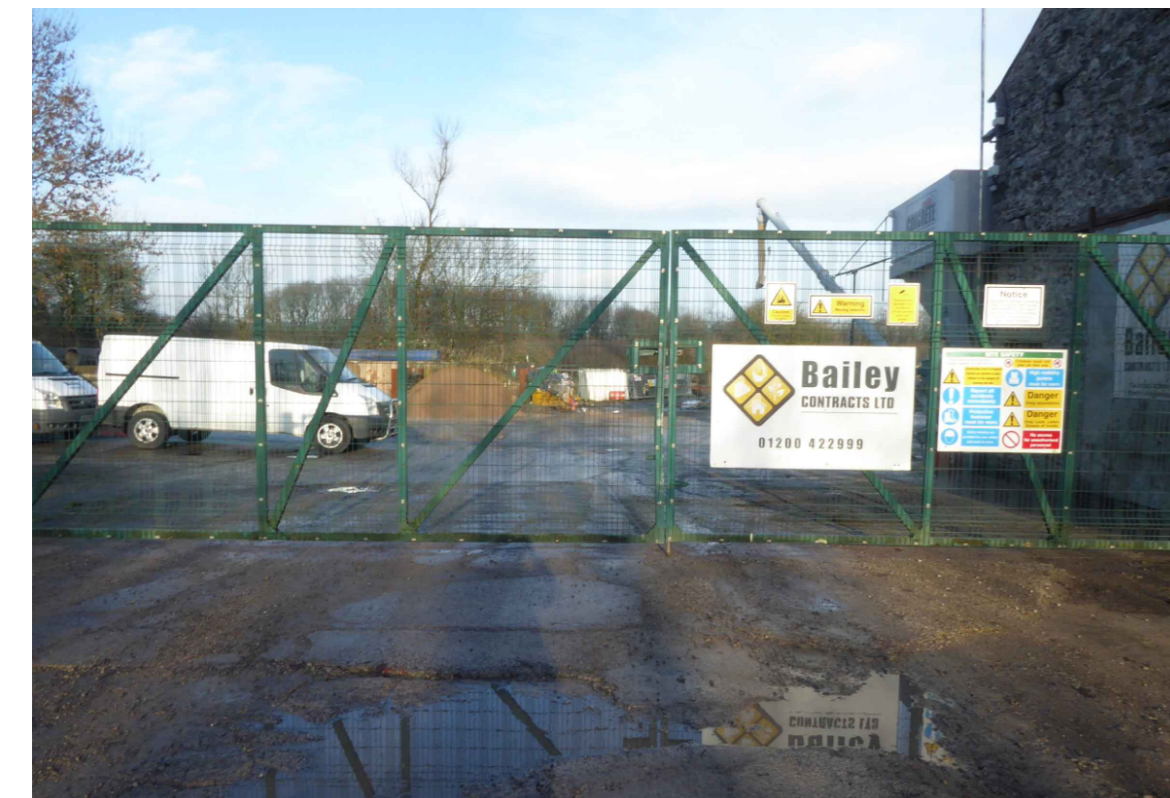
Security Fence and Gate
