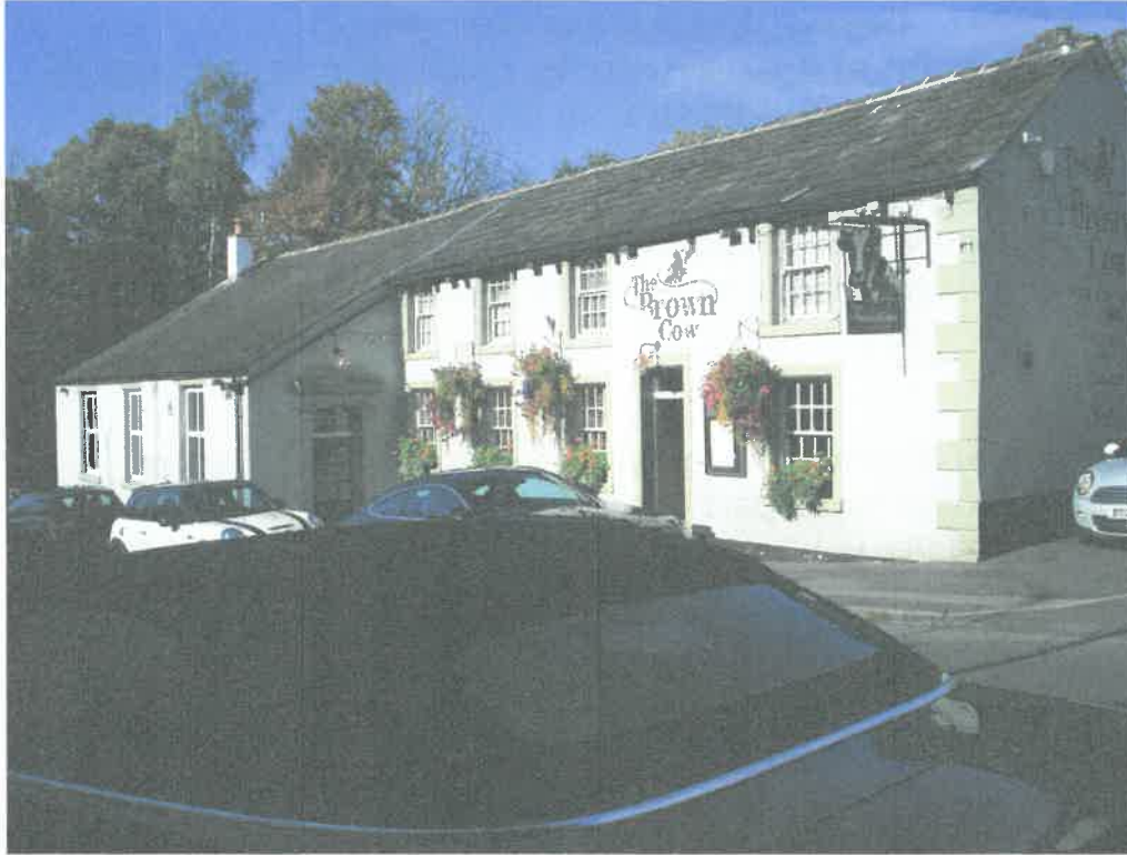
Front Elevation onto Bridge Road
