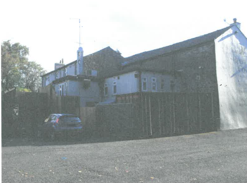
Rear / Side Elevation from car park looking towards kitchen
