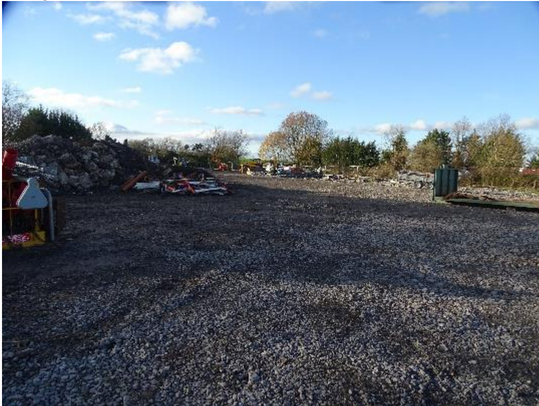
Looking across the site
