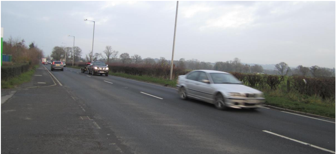
1 View north along Longsight Road carriageway bordered by high hedges.
