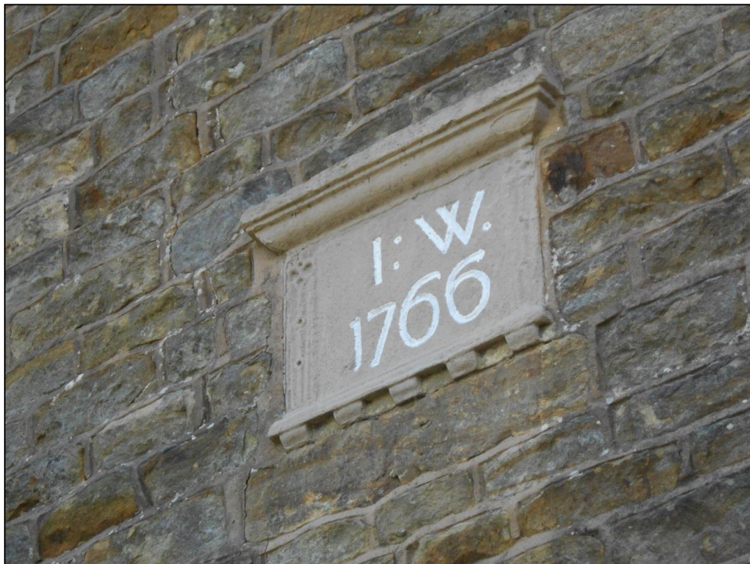
PL00: Date stone present to the front west facing elevation of the building.
