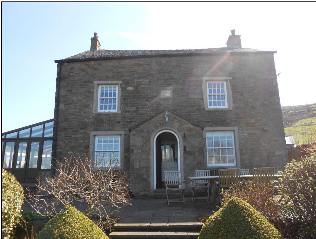
PL00: View of the front of the building from the west
