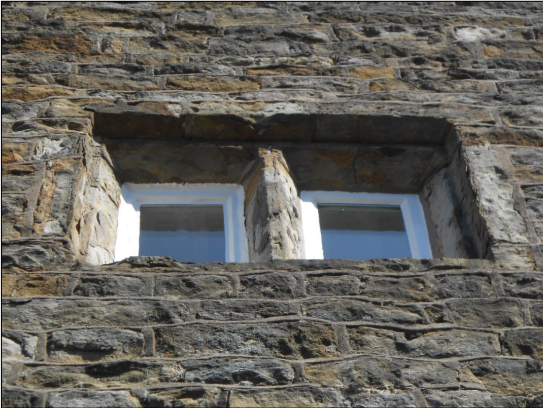
PL00: Window present to the second floor with straight chamfered mullion and jambs.
