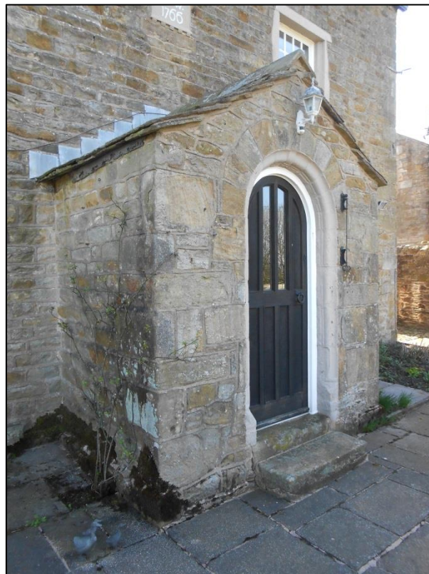
PL00: Front entrance porch to the west elevation of the building
