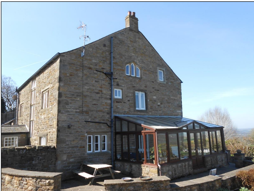
PL00: View of the building from the north
