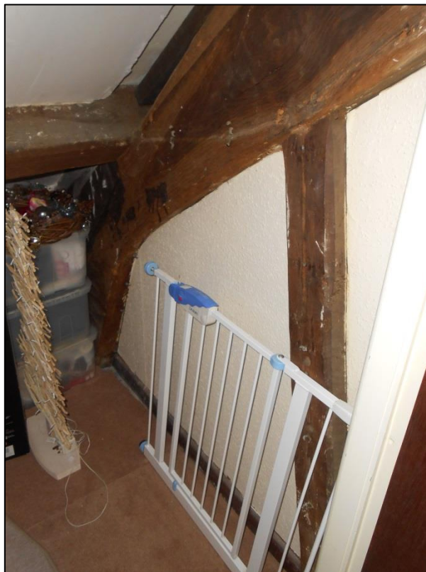
PL00 Upper cruck noted to the attic / second floor of the building
