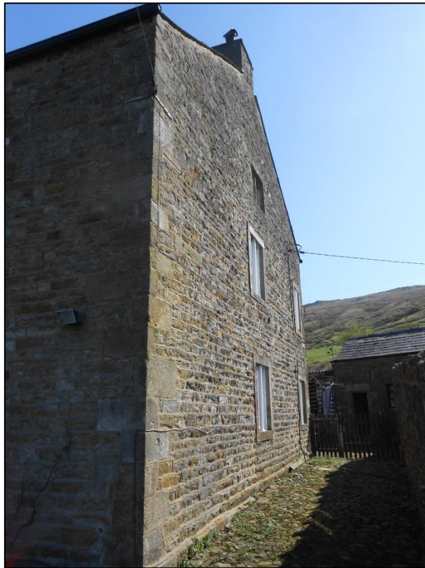
PL00: South facing elevation of the building
