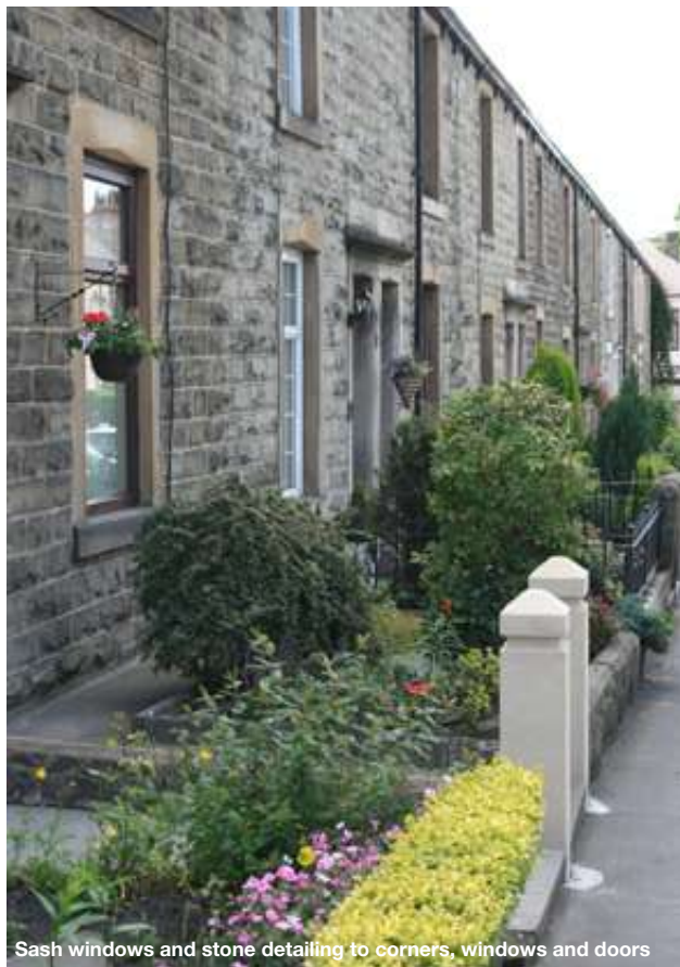
Stone terraced housing with bay window detail
