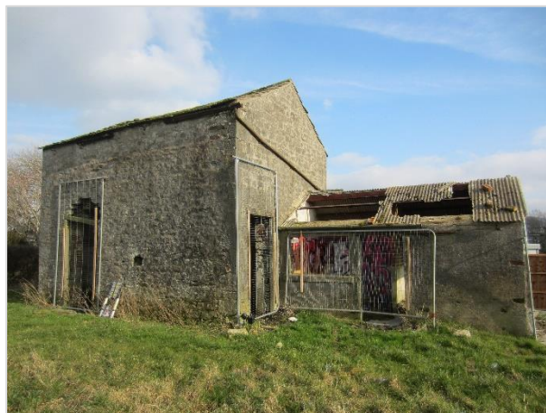
Insert 1: West and south elevations of the stone barn
