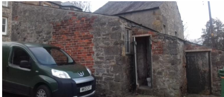
Side elevation showing door to store and lean to porch.
