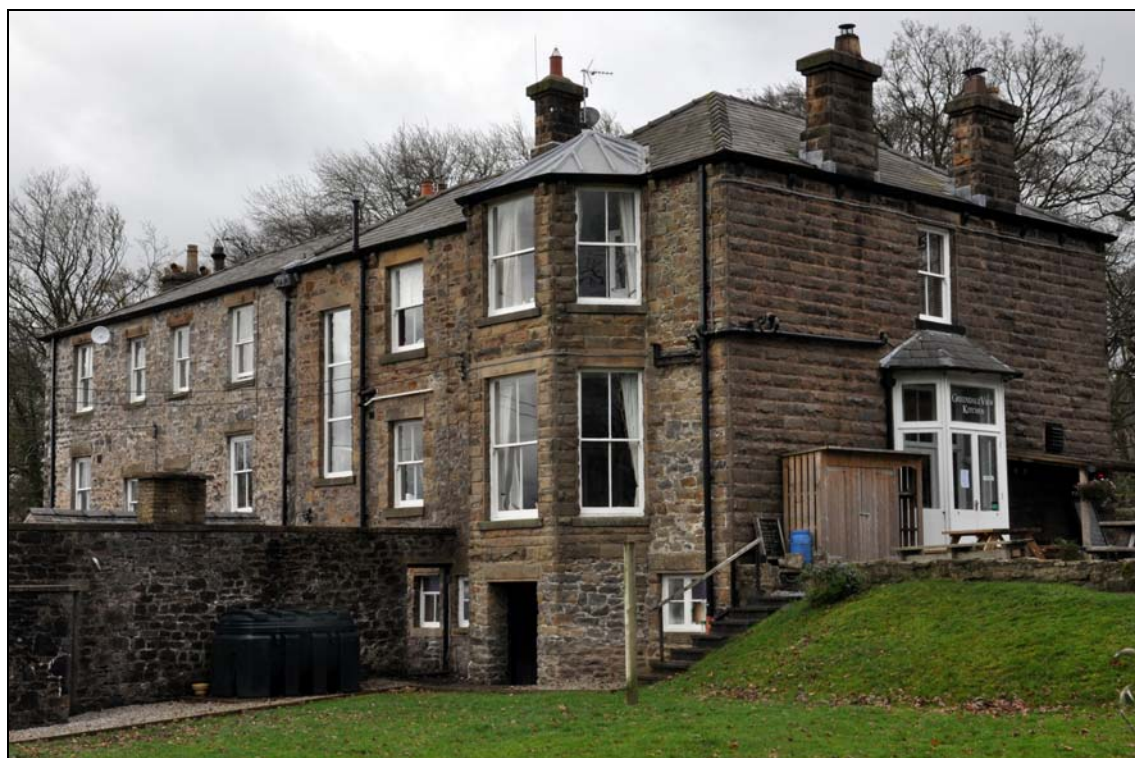
Photo 3: Temperance hotel addition, looking south-east
