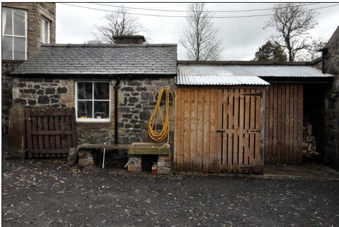
Photo 8: East side of wash house
