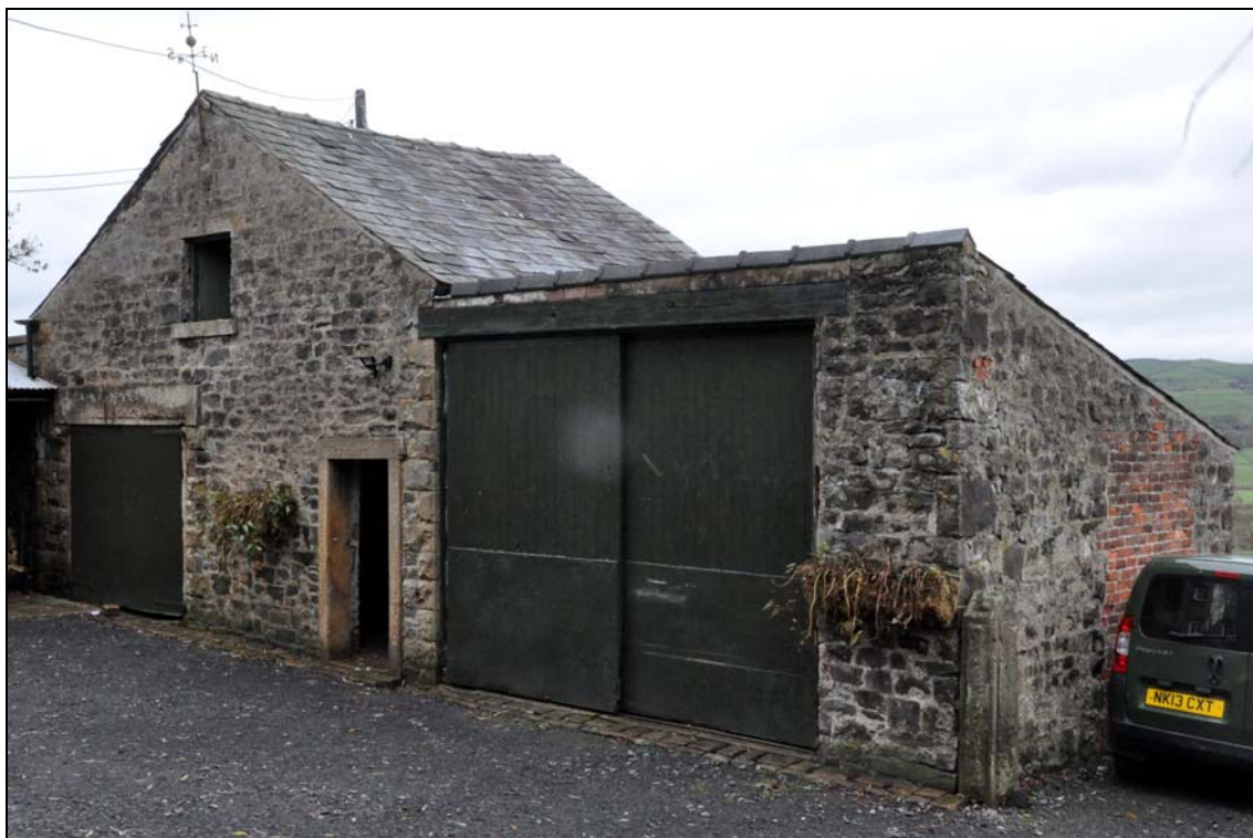
Photo 4: Two storey trap house and stable, with later trap house or motor garage to right
