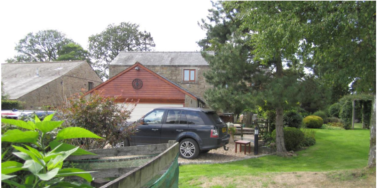
2 East elevation with garage and fir tree
