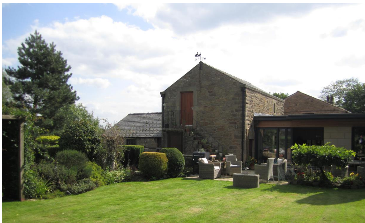
1 North elevation of outbuilding with external staircase.
