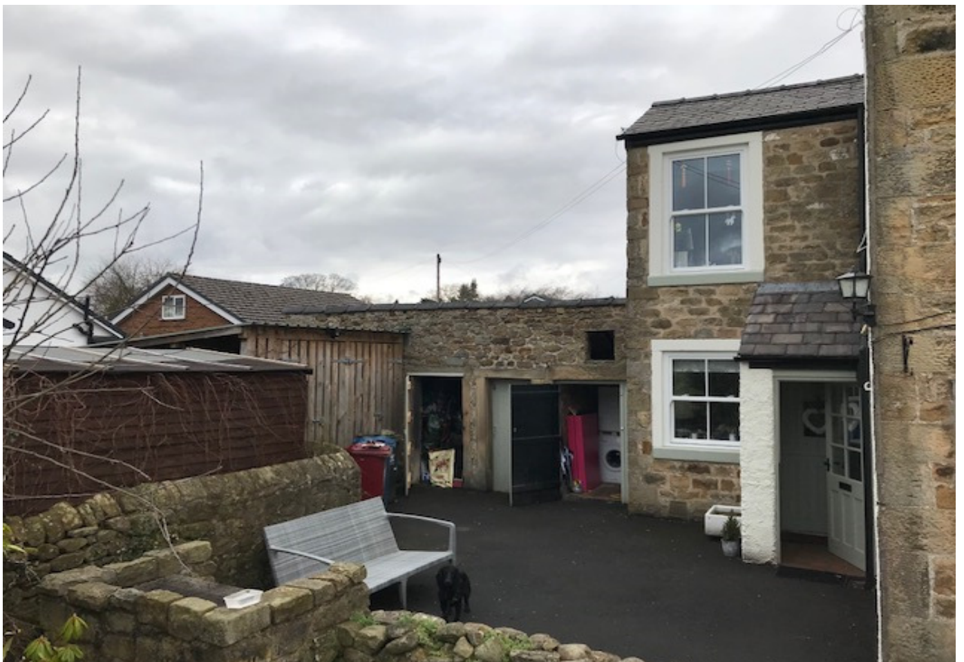
Views of the property from the north and south
