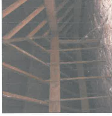
Photo 6: Interior of loft space showing roof construction
