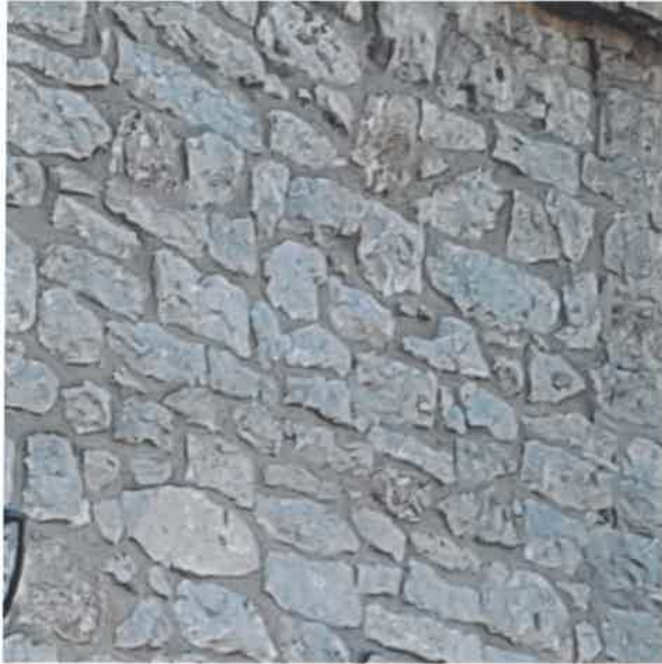
Stone to be used for porch
