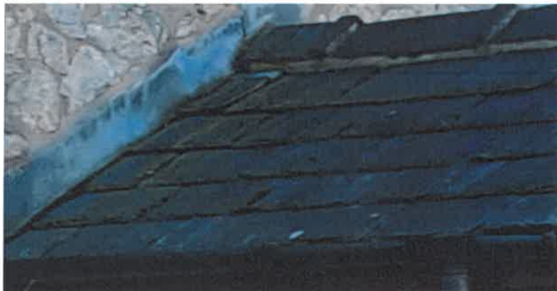
Slate to be used for porch roof
